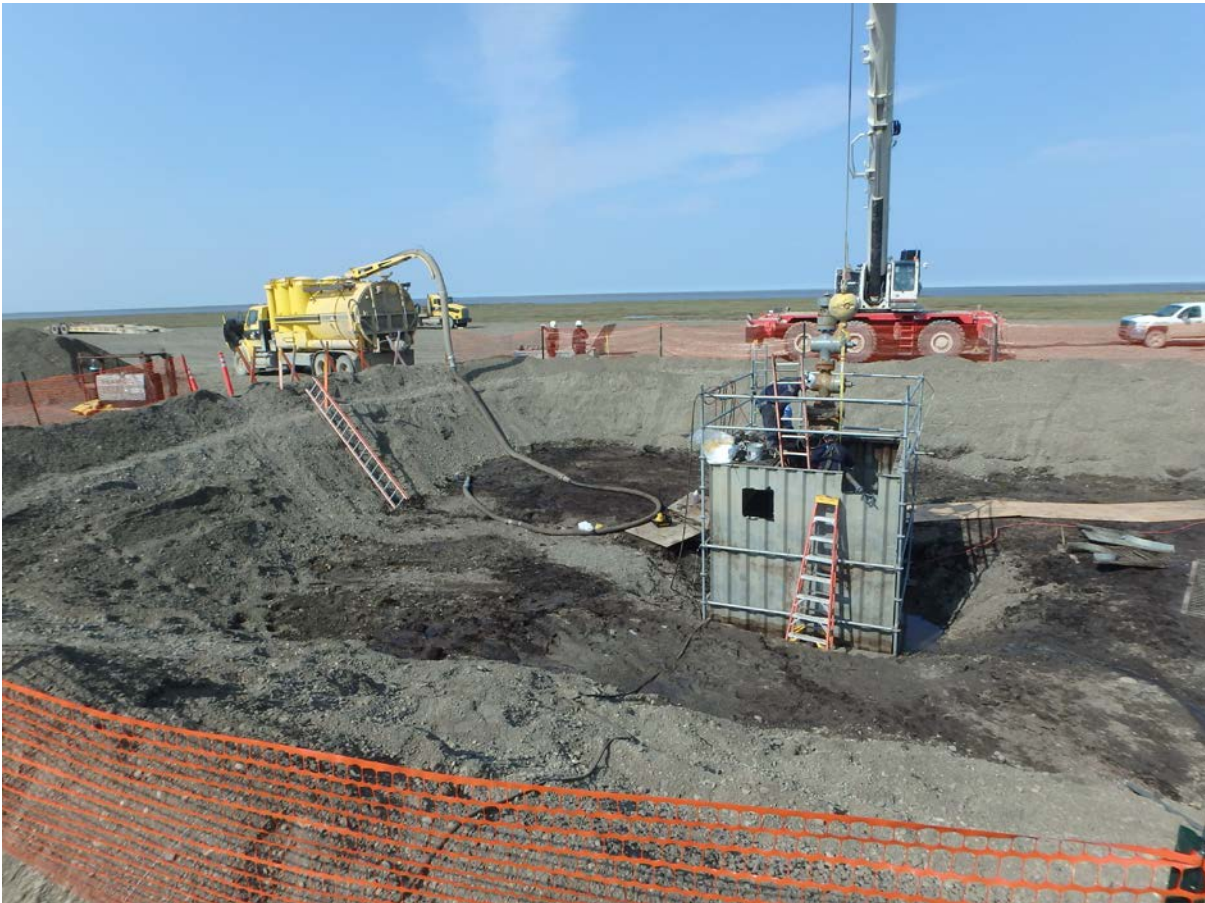
Nuna Pad 2 Cellar with Super Sucker on site during the repair of the outer annulus flange. (Photo credit Wes Ghormley, ADEC, July 13, 2017).
