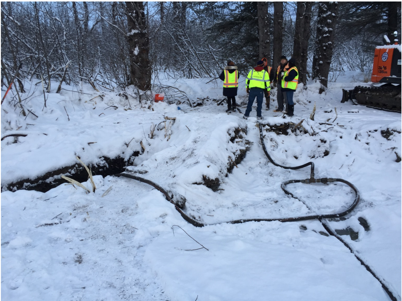
Fuel recovery operations, 2/26/2018 (Photo/ADEC). (Photo by ADEC)
