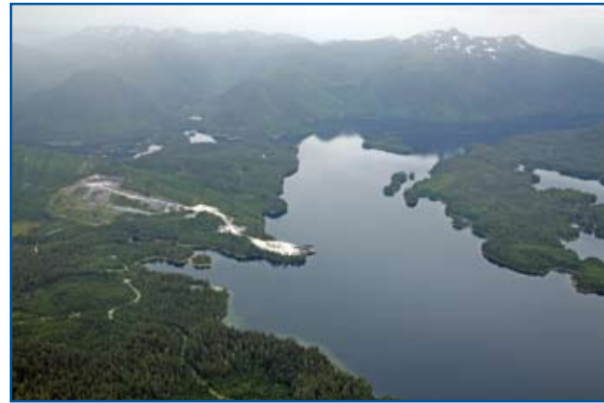
Admiralty Mine dock viewed from the north.
