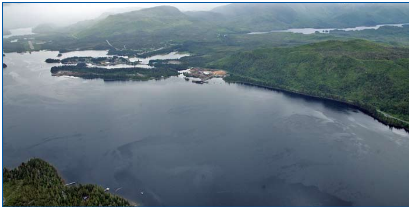
Klawock D-02-03, Mill Dock, & D-02-04, AML Dock viewed from the southwest.
