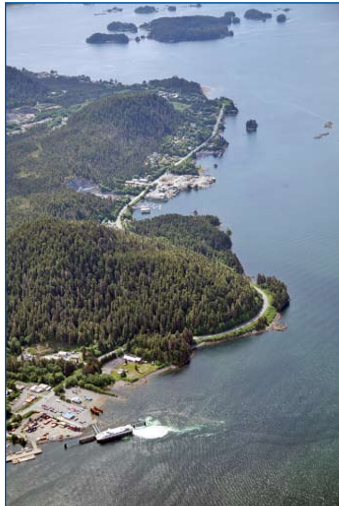
Sitka Ferry Terminal and Samson Tug Dock viewed from the northeast.
