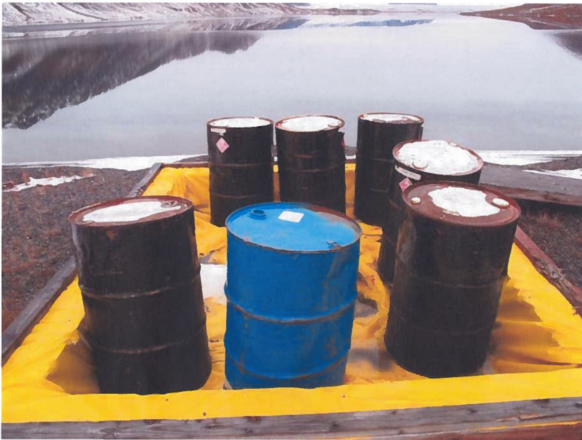
Photograph 4. Designated drum staging area surrounded by portable foam sided berm (69°18'18"N latitude, 145°01'53"W longitude)
