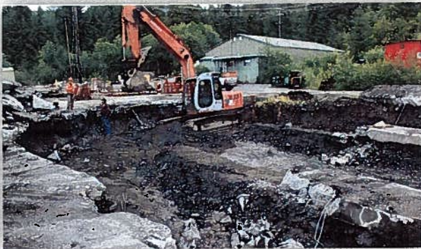
Figure 7: View on 7/20/12- looking toward the north end of the green chain/ sorter line after the former 'action pack' foundation had been removed for continued excavation of contaminated soil
