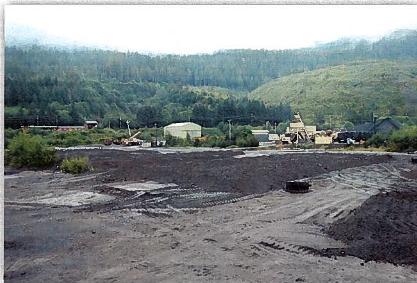
Figure 17: July 23 view showing 4 of the 5 Biocells that have been turned and tilled
