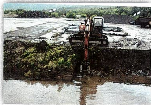
Figure 5: 6/30/12 excavation of oil/water separator
