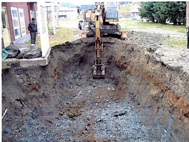
Dense gray sandy/silt/clay layer between eight and ten feet BGS in the main UST excavation.
