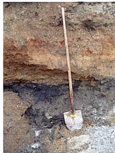
Dense gray sandy/silt/clay layer between eight and ten feet BGS in the main UST excavation.
