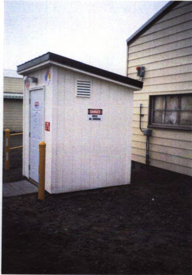
ABOVEGROUND STORAGE TANK (AST) 19-D-5 SITE AFTER EXCAVATION HAD BEEN BACKFILLED AND A VEHICLE FUEL DISPENSER SHED RELATED TO UNDERGROUND STORAGE TANK 19-D-104 CONSTRUCTED, VIEWING SOUTHEAST.
