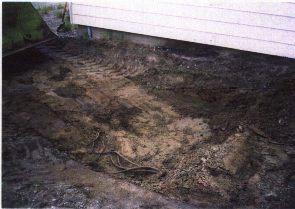
EXCAVATION BELOW FORMER LOCATION OF AST 19-D-5, VIEWING SOUTH.
