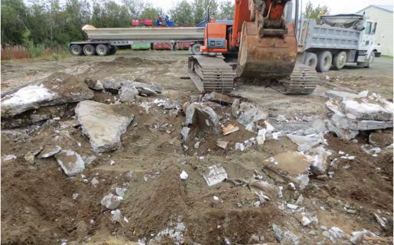
Photo 9: Concrete pad prior to its demolition; facing southeast (September 2, 2014).
