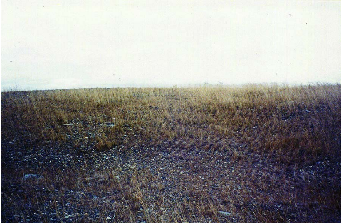
Photograph 5 - View of east side of landfill cap, looking west (20 Sep 2001)
