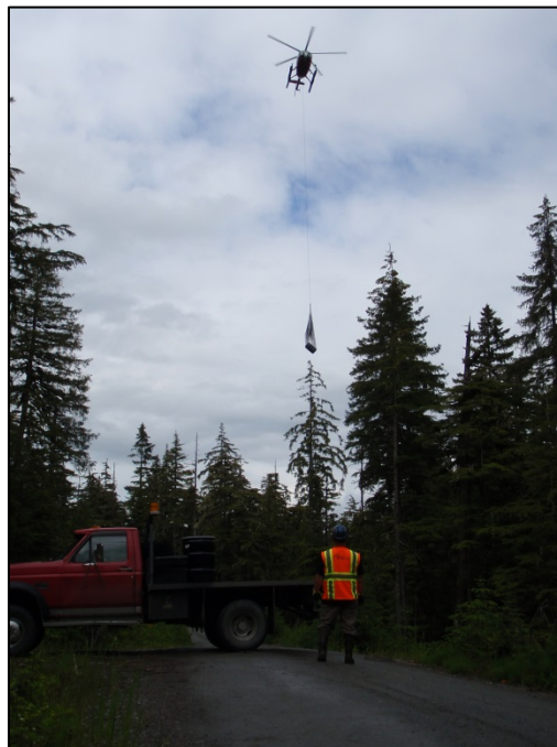
Photograph 4: Transporting 55-gallon drums from site to nearby road via helicopter.
