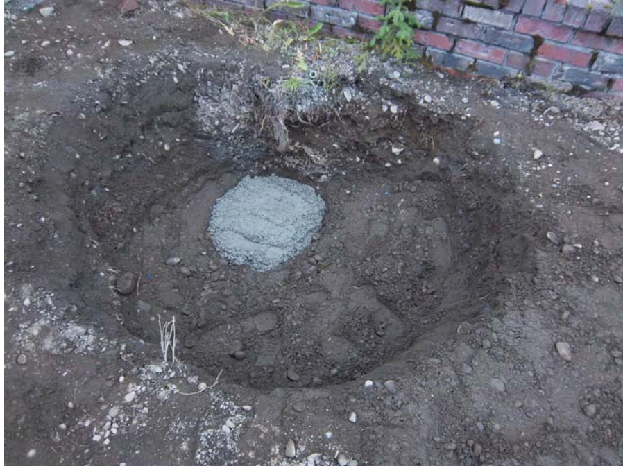
PHOTO 4 – Potable water well decommissioning complete; hole backfilled with native soil to grade.
