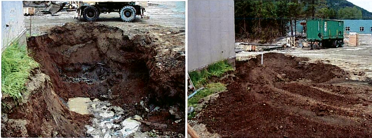
Stained grey soil layer in the north wall and groundwater monitor well emerging from clean backfill soil.
