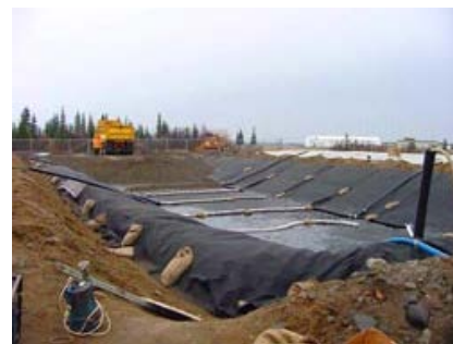
This biocell used to treat petroleum-contaminated soil in King Salmon is a large pit lined with material which prevents contamination from passing through it while the soil is being treated. (DEC photo)
