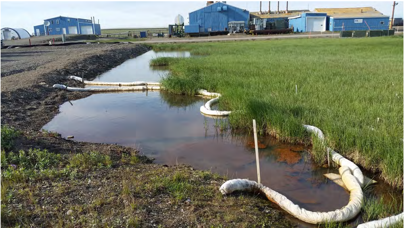
Photo 3: Sorbent booms at the liner gap. Photograph faces north-northwest.
