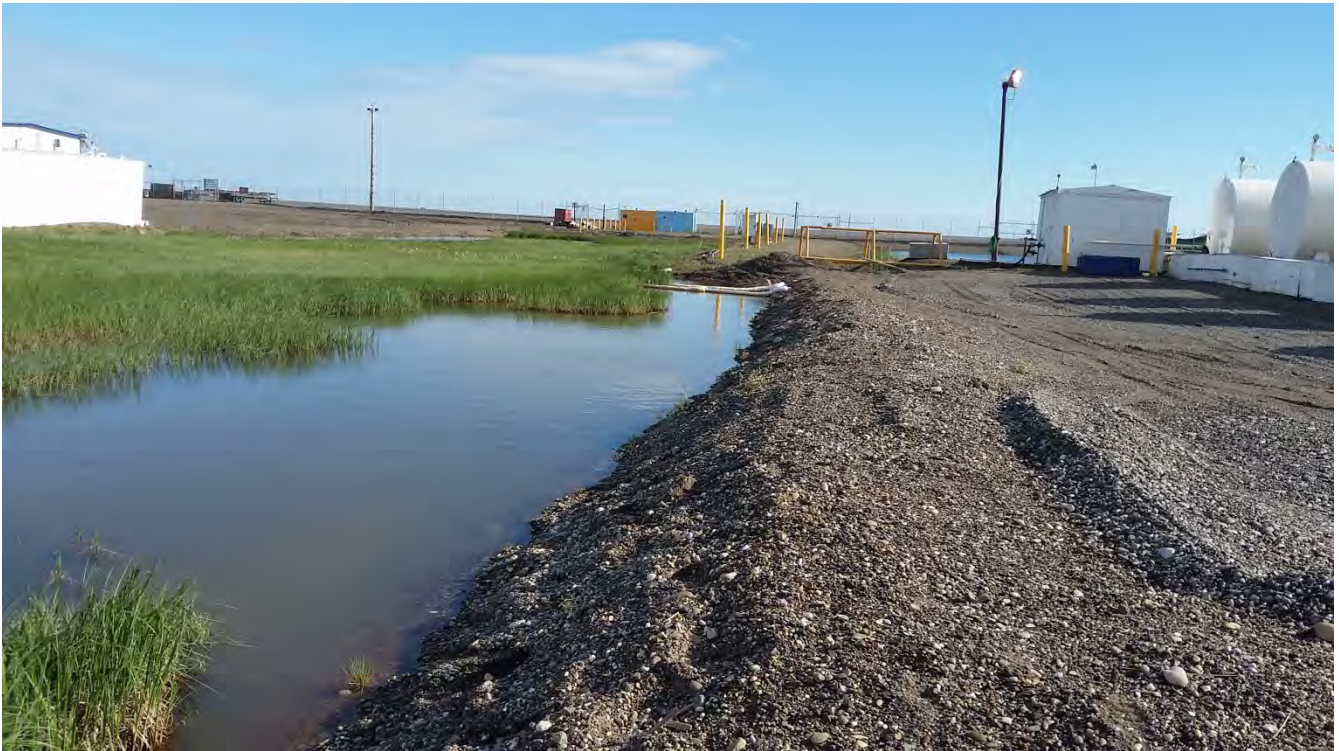
Photo 2: Northeast edge of the north pond. Photograph shows well-formed berm along pad edge. Photograph faces east.
