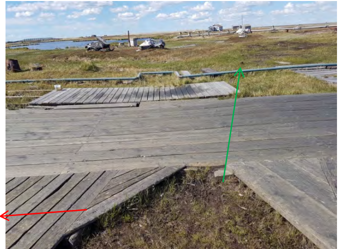
Photo 2: Looking North - View of historic boardwalk and pipeline spill area. BH06 (red arrow) was to the left of photo on the other side of the small boardwalk. The green arrow points to BH05.
