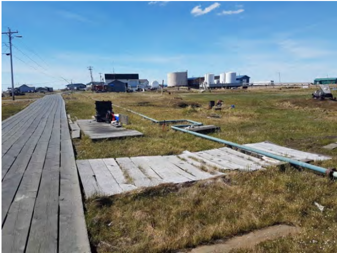
Photo 1: View of the pipeline spill area. Historic boardwalk is visible with equipment placed on top.
