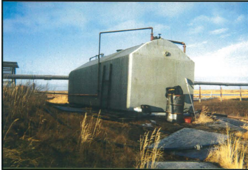
Village: Kwigillingok ADEC Site Number: 2 Site Name: Kwig Incorporated, Washeteria Direction: NE Description: 10,000-gallon AST on east side of the Washeteria.
