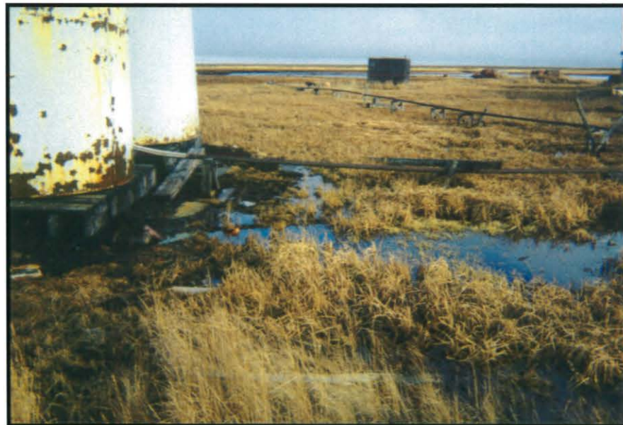
Village: Kwigillingok ADEC Site Number: 3 Site Name: Old BIA School, LKSD Direction: E
