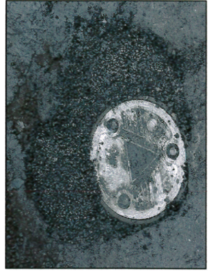
MW#12 INSTALLED, PROTECTIVE COVER IN PLACE
