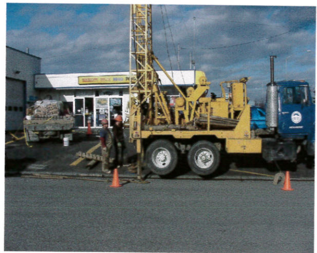
Installing Monitoring Wells May 2002
