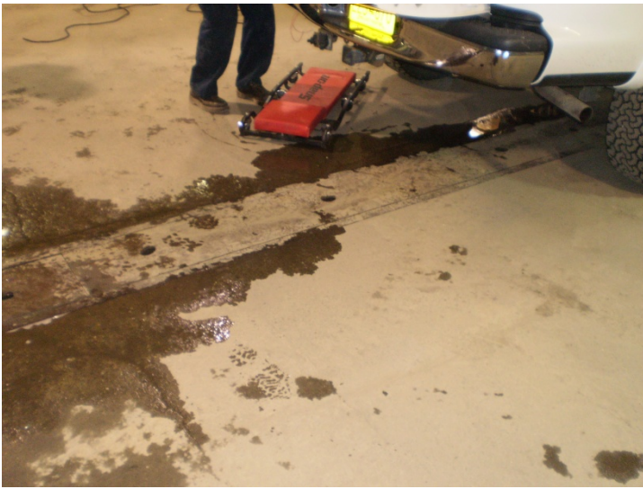
Photo 7. Floor Drain in Western Garage Area
