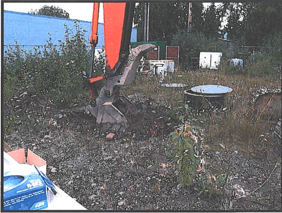
5. Test Pit 3 excavation in progress.
