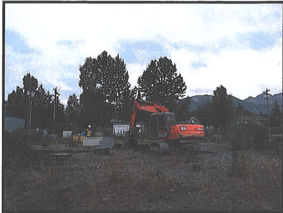
3. Test Pit 2 excavation in progress.
