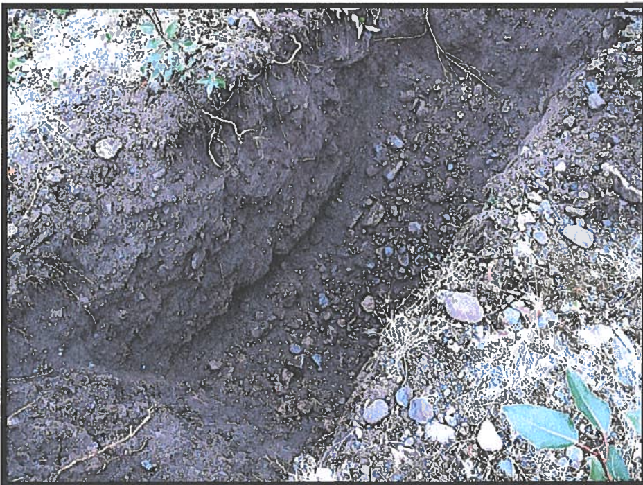
6. Test Pit 3 completed excavation.
