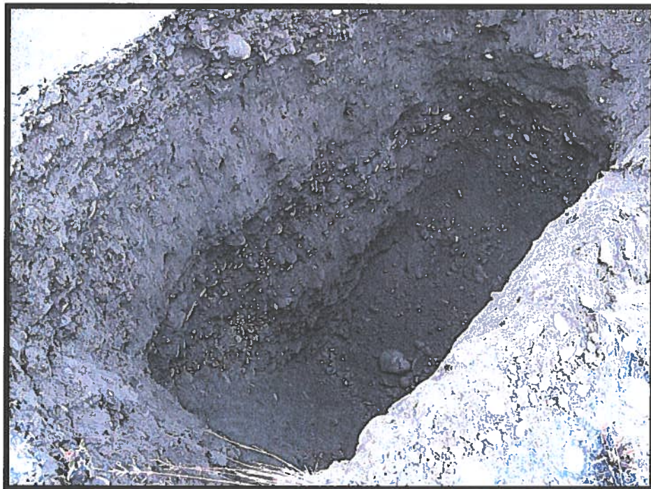
4. Test Pit 2 completed excavation.
