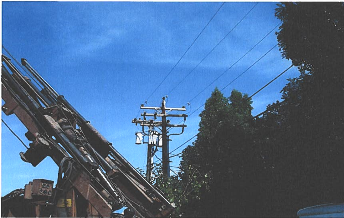
3. MW-1 Due to the close proximity of overhead power lines, the drill rig's mast could not be raised to pull the well.
