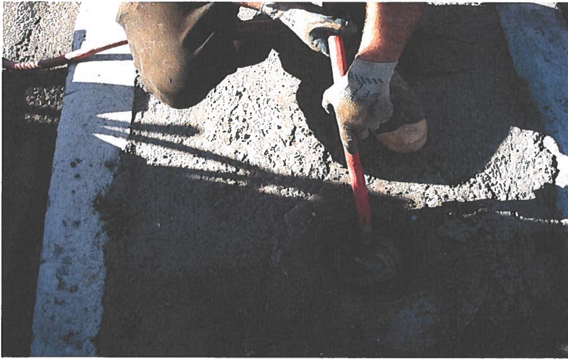
17. MW-7 Topping off the well bore with grout.
