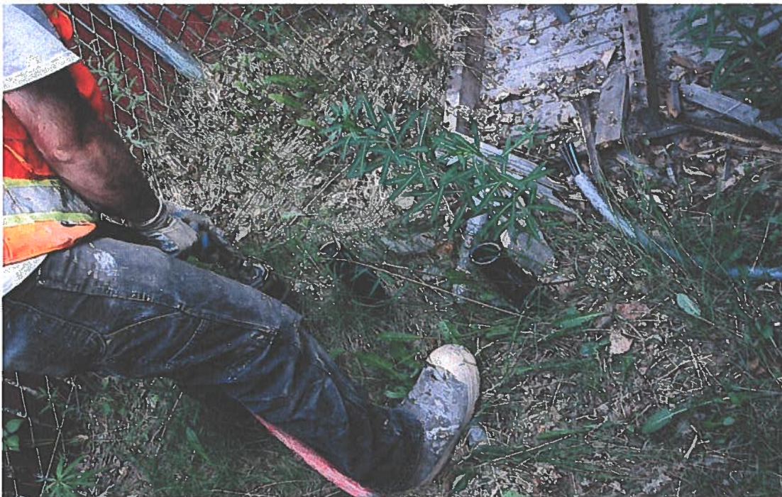
42. Pressure grouting the SVE lines next to the Remediation Shed.
