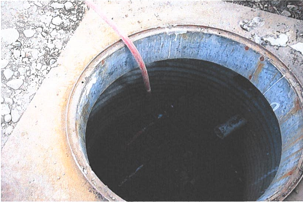
51. VCS-1 Pressure grouting air line from the vault to Remediation Shed.
