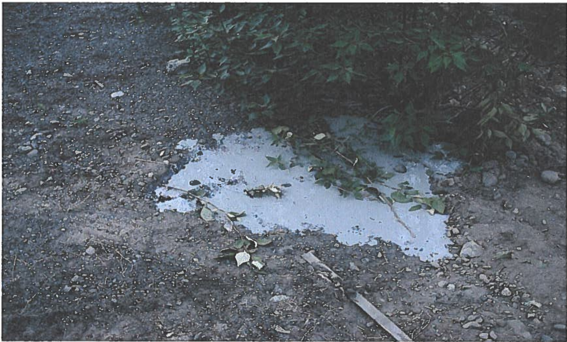
46. SVE-2 Location of horizontal well where grout daylighted by pressure.
