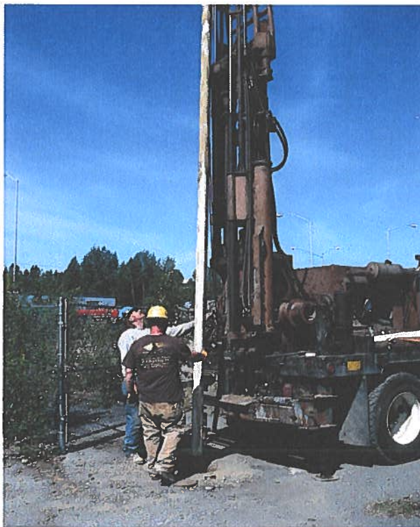
17. MW-7 Topping off the well bore with grout.
