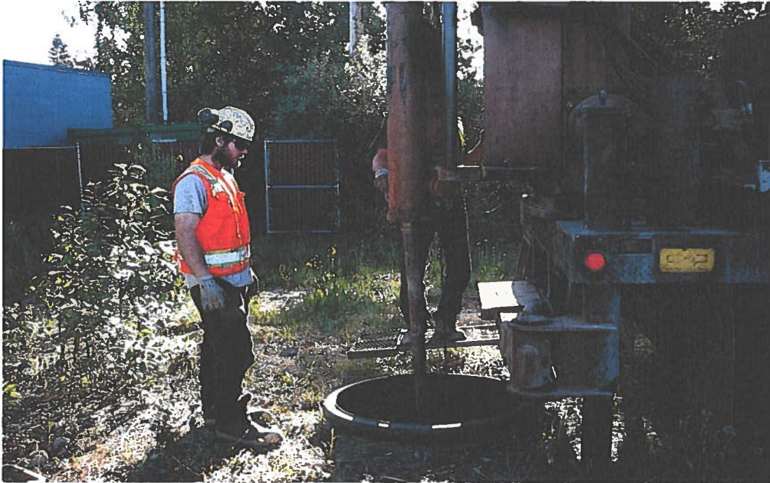
39. CW-3 Breaking out the bottom of the well casing.
