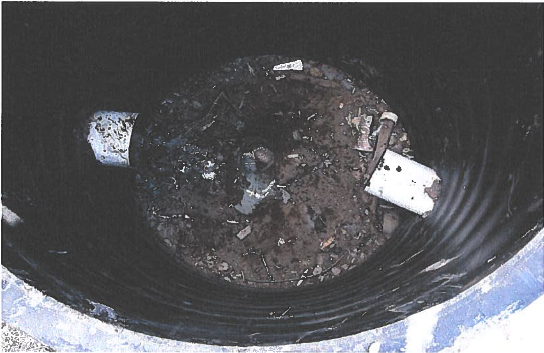
23. MW-14 Former well topped off with grout.
