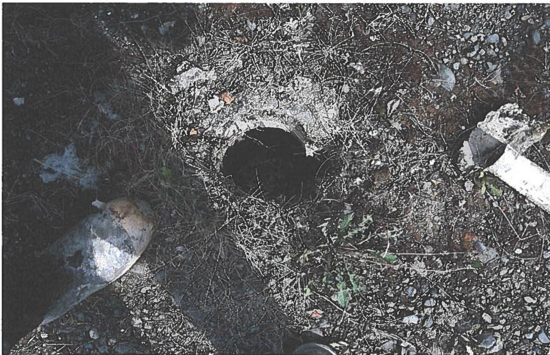
30. MW-16 Topped off well with grout.
