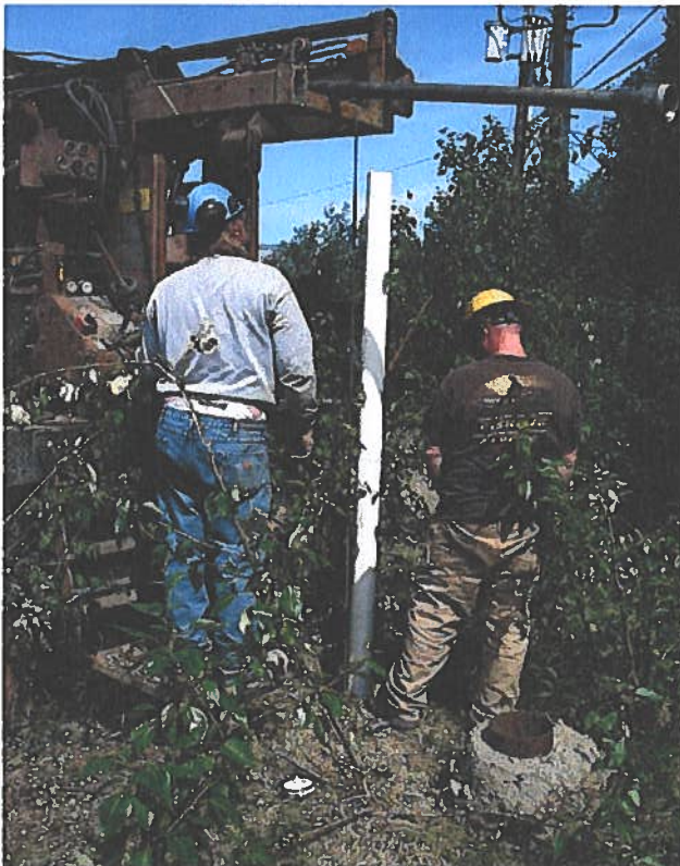
3. MW-1 Due to the close proximity of overhead power lines, the drill rig's mast could not be raised to pull the well.
