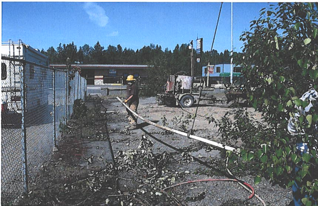
32. MW-17 Walking out well casing, grout line in the foreground.
