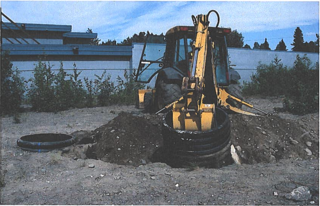
24. MW-14 Removing the protective vault; Circulation Well CW-2 vault to left.
