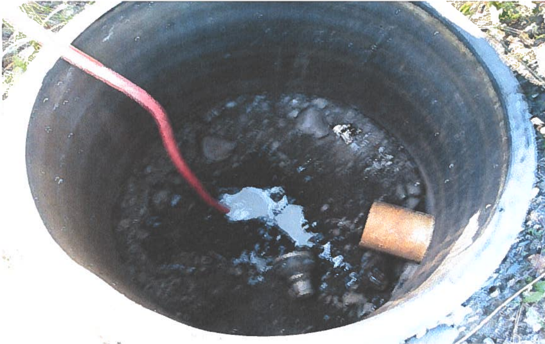
41. CW-3 Grouting the former well.
