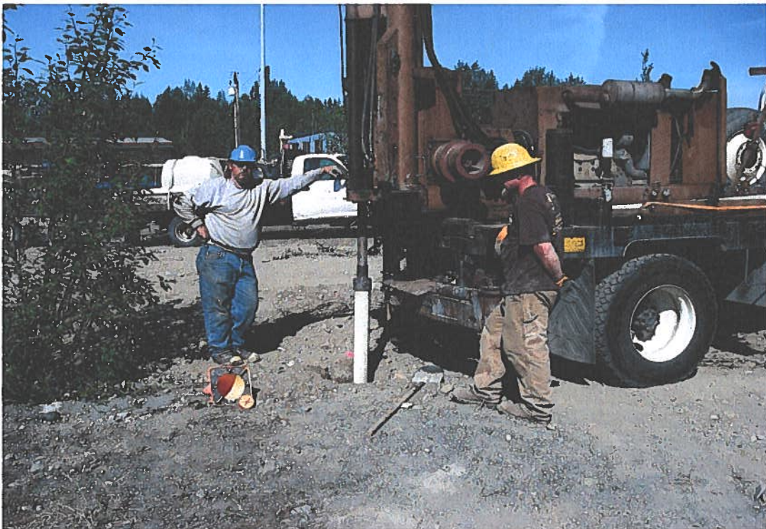
44. SVE-1 Pulling well casing with threaded bell cap .
