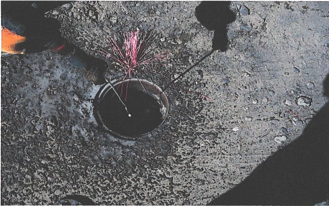
19. MW-8 Topping off the well bore with grout.
