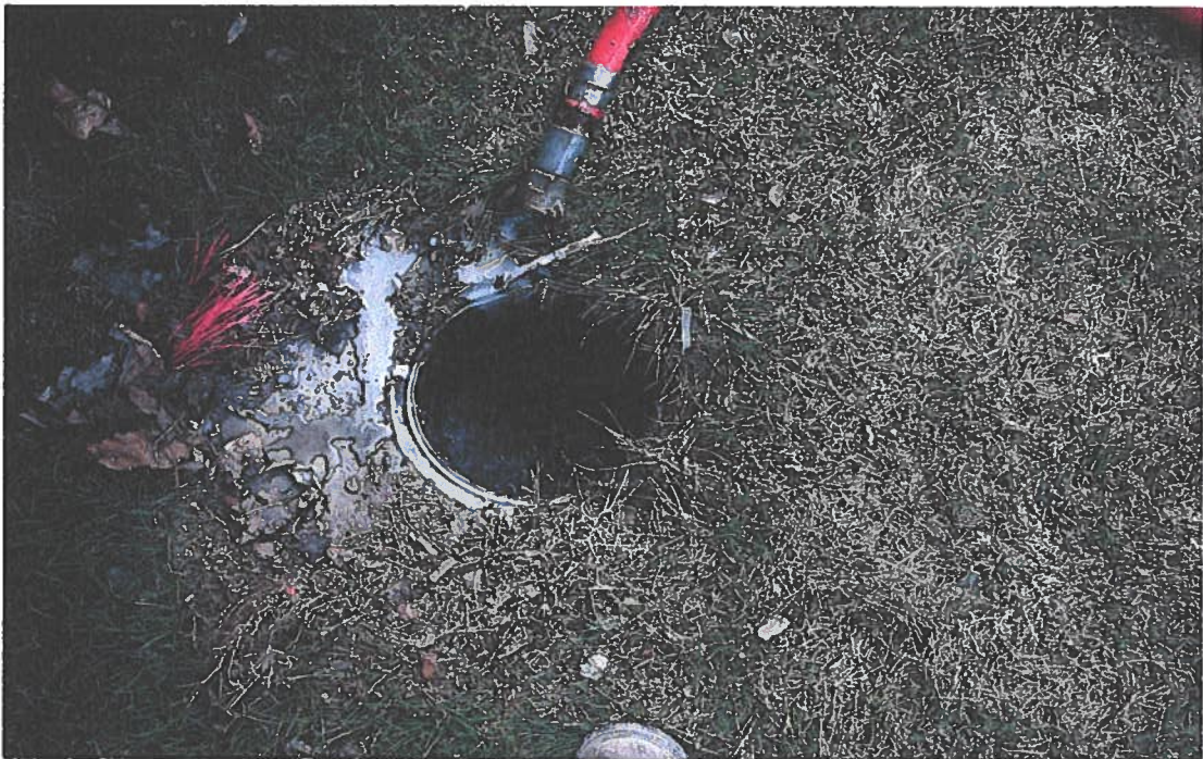
7. MW-4 Stabilized grout in bore hole.
