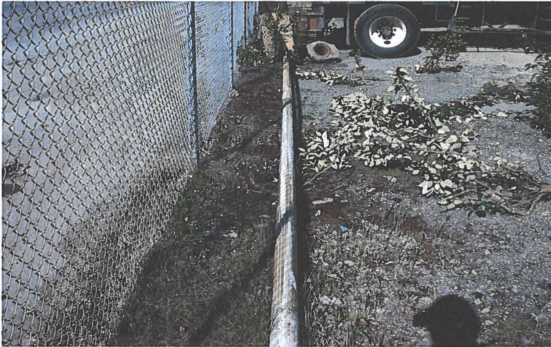
5. MW-3 Pulled well casing.
