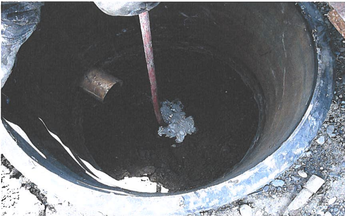
38. CW-2 Former well void filled with grout.
