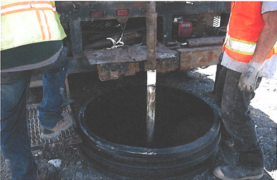
21. MW-14 Pulling the well casing with a taper tap.
