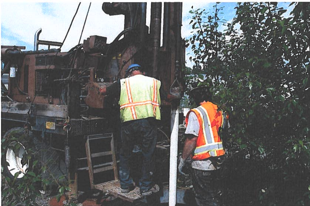
54. VSC-1 Pulling well casing.
