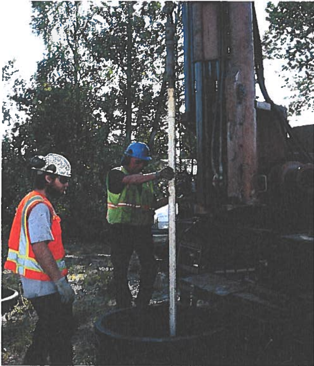
25. MW-15 Pulling the well casing with a taper tap.
