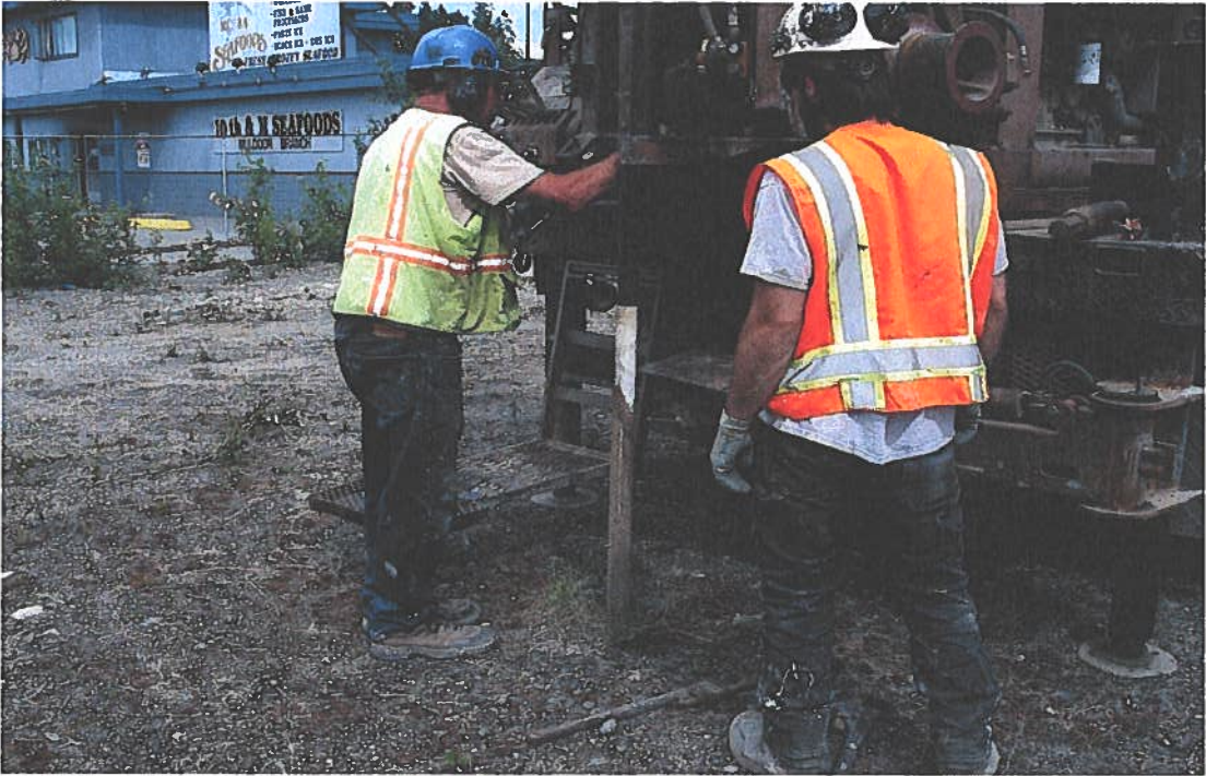
28. MW-16 Pulling the well casing with a taper tap.
