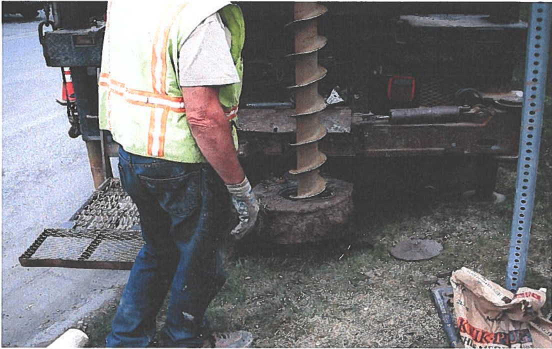
9. MW-4 Removing cement encased protective vault with drill rig's auger.
