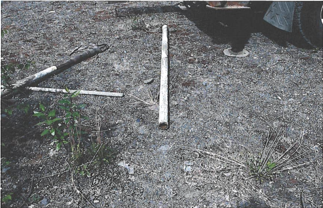
29. MW-16 Removed well casing with bottom broken out.
