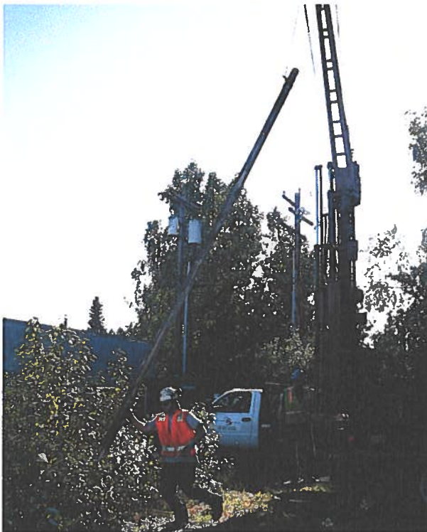
39. CW-3 Breaking out the bottom of the well casing.
