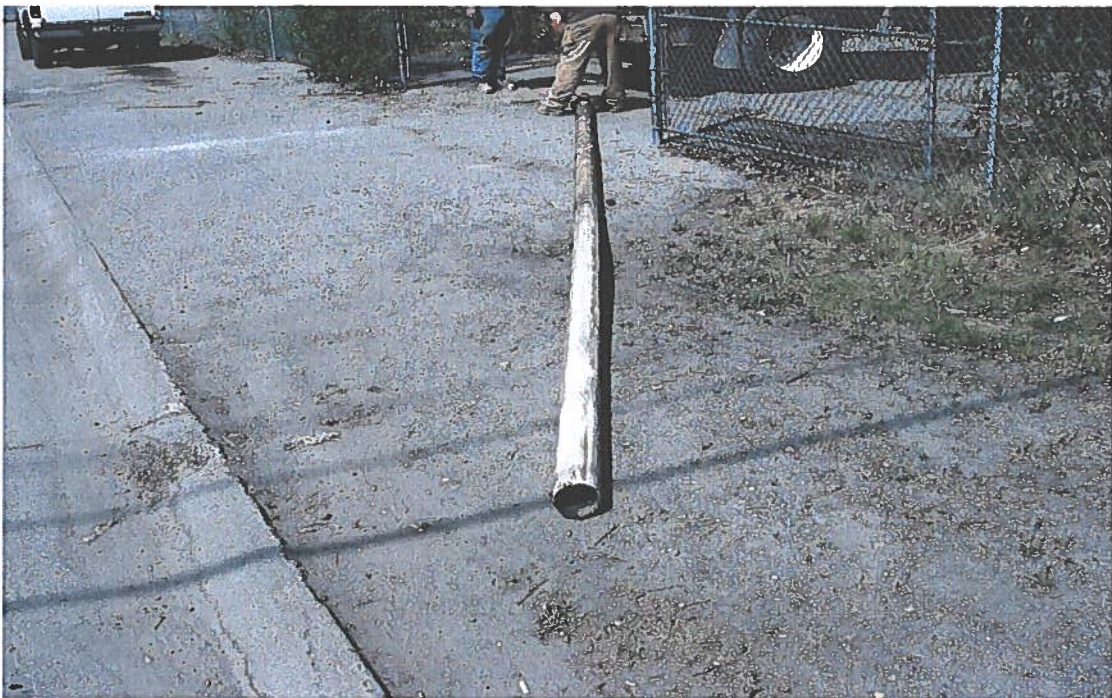
20. MW-8 Pulled well casing with bottom knocked out.
