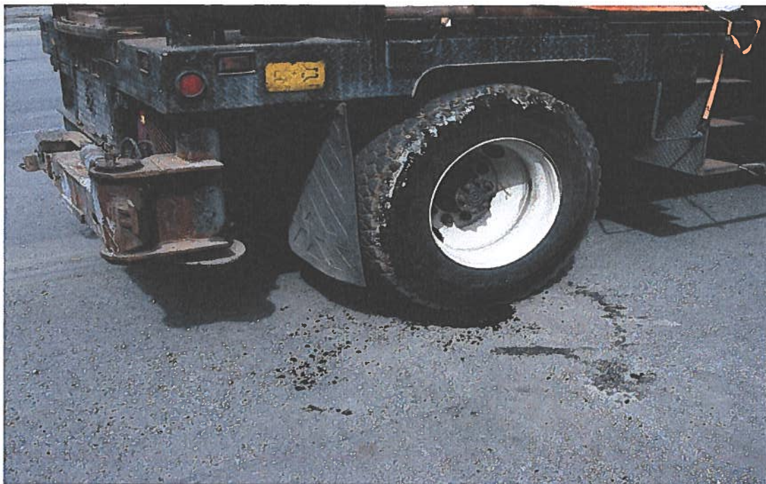
12. MW-5 Using the drill rig to compact the asphalt cold patch.
