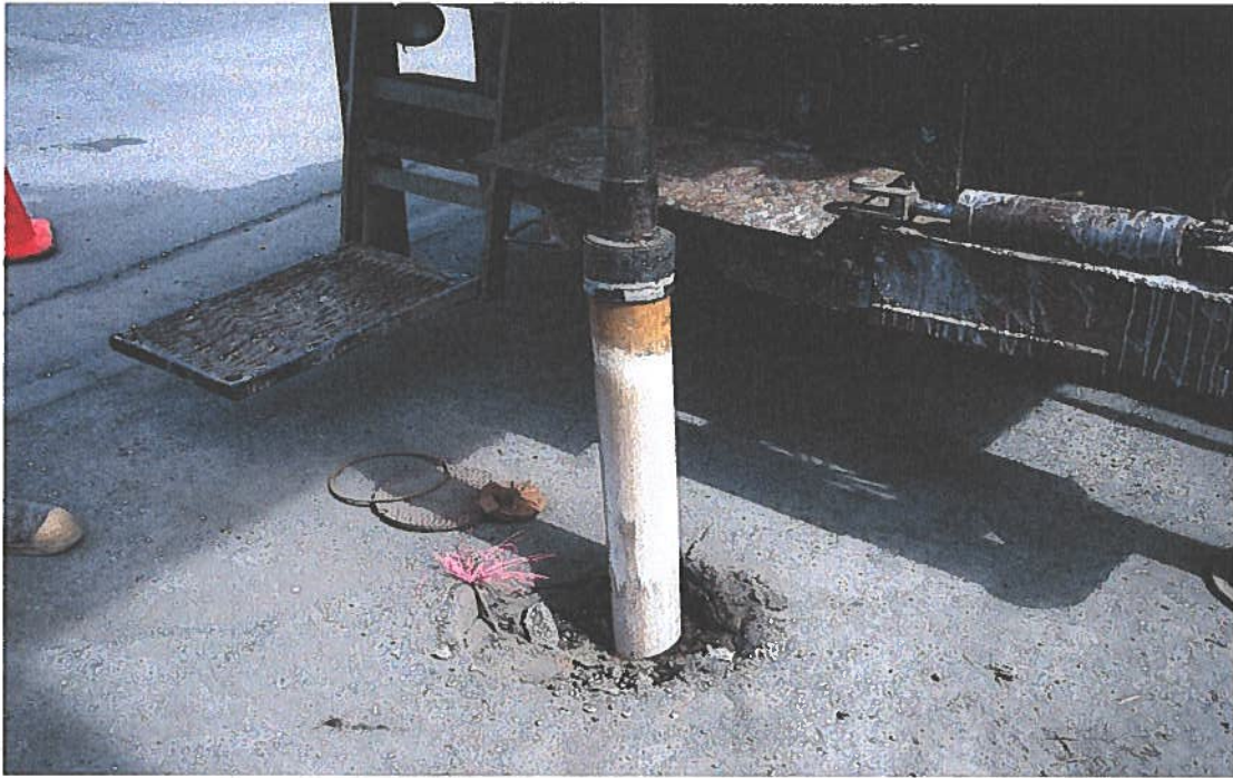
13. MW-6 Pulling the well casing with a threaded bell cap .
