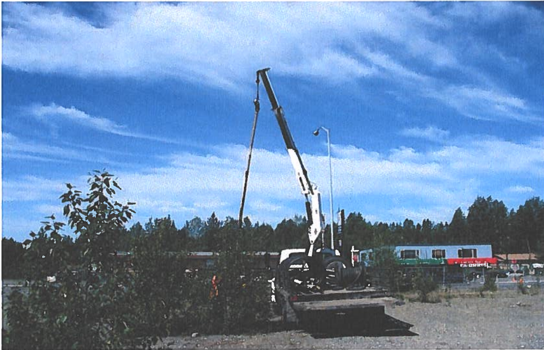
53. VSC-1 Pulling eductor piping with a boom crane.
