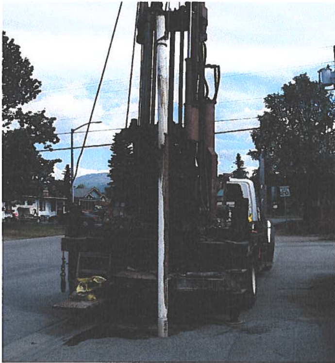
11. MW-5 Pulling the well casing.
