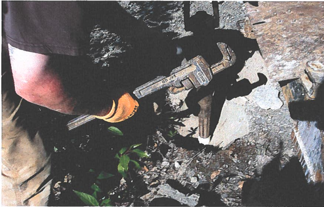
31. MW-17 Driving a taper tap in preparation of pulling.
