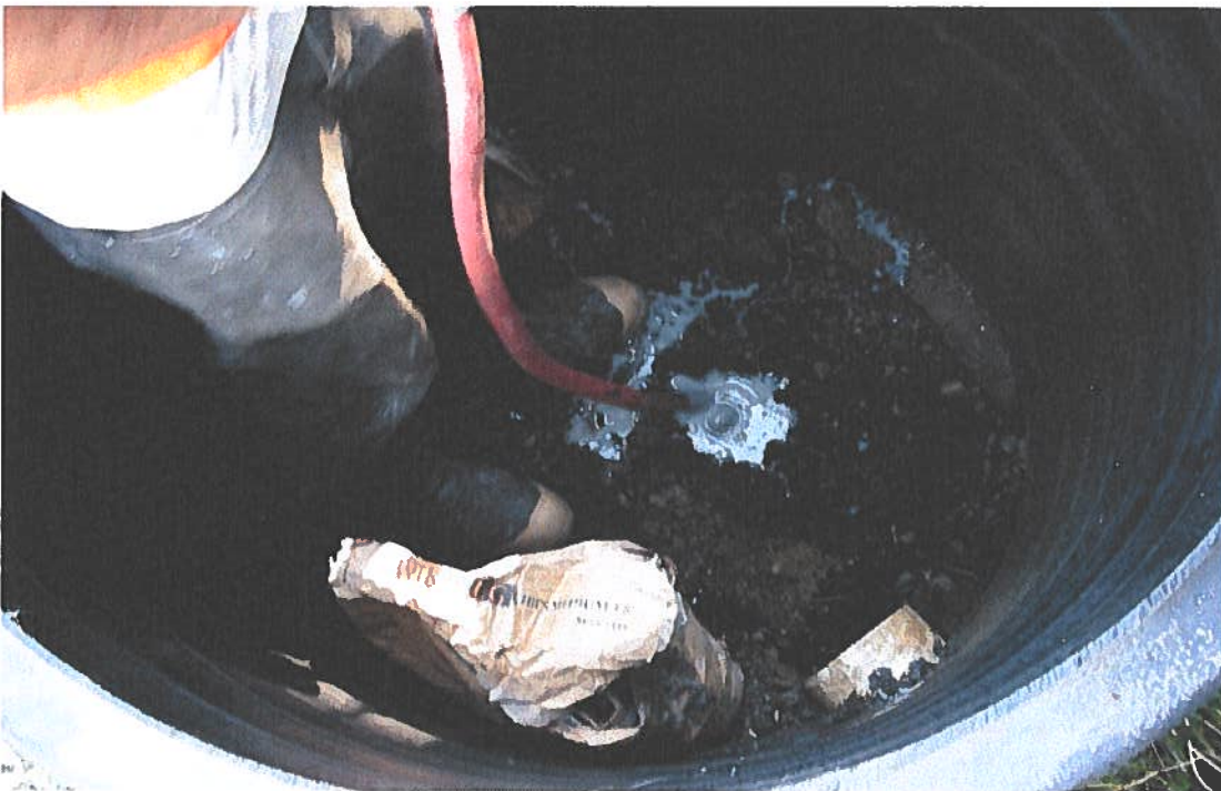
26. MW-15 Topping off the well with grout.
