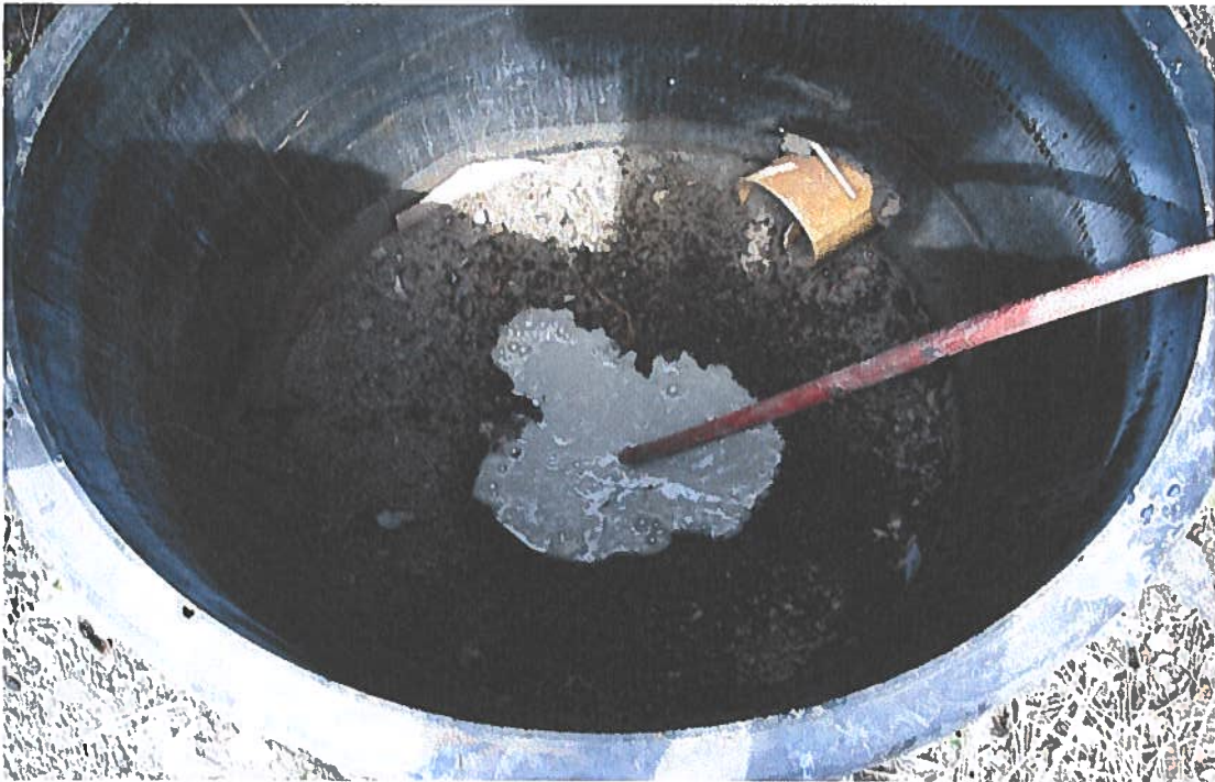
35. CW-1 Grouting the former well.
