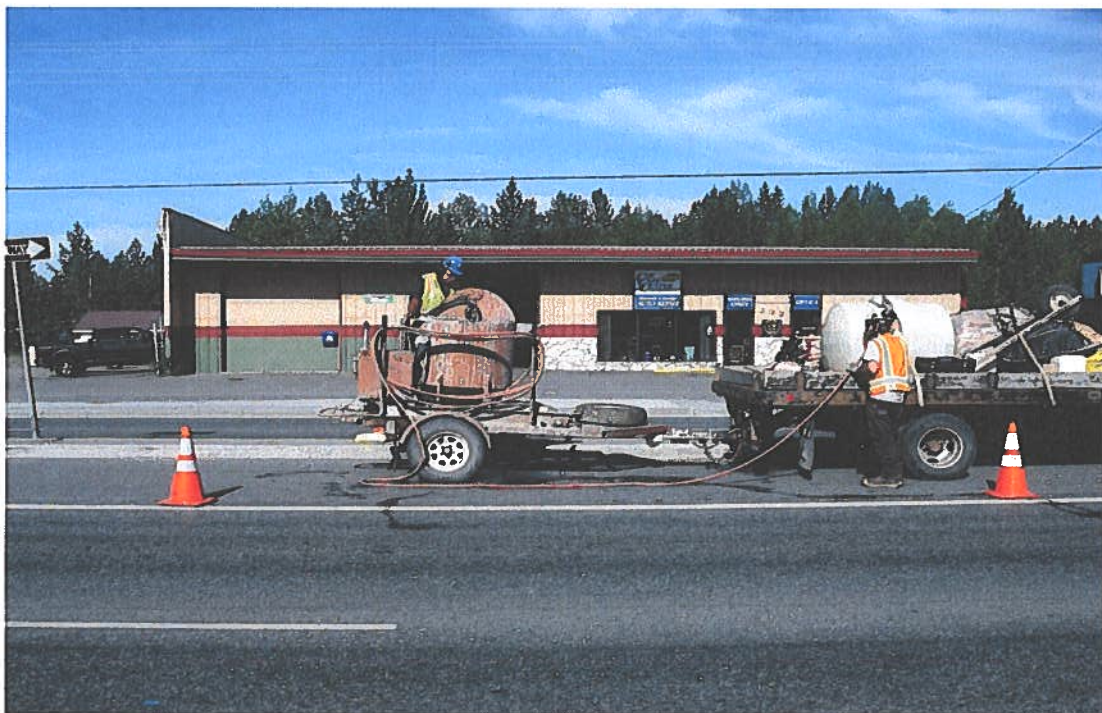
16. MW-7 Showing the grout plant in position .
