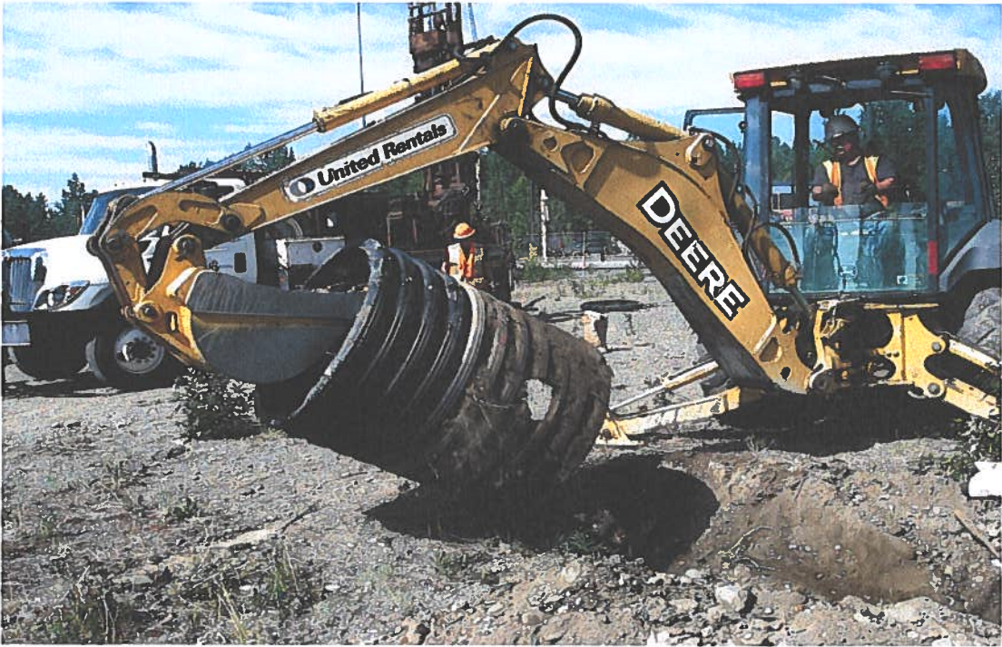
27. MW-15 Removing the protective vault and associated conduit.
