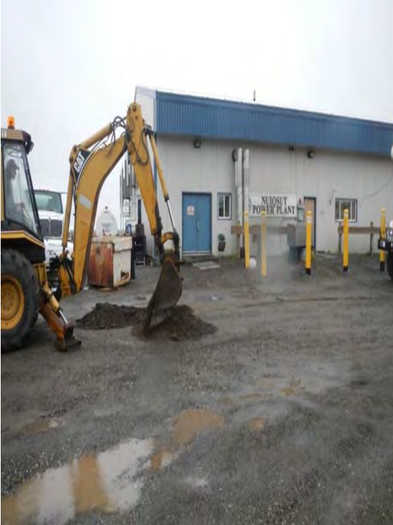
Photograph 5. Excavating Test Pit #2 (Sample Location #17). Looking toward Nuiqsut Power Plant Building.
