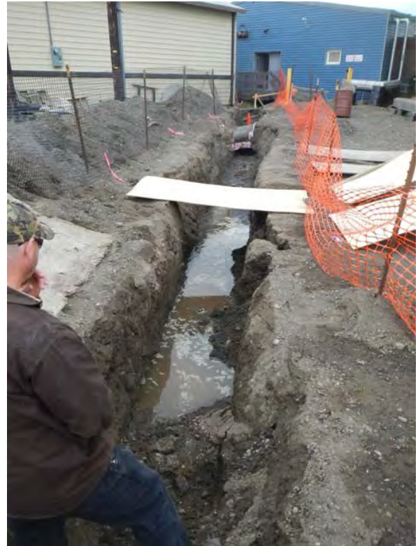
Photograph 2. Trench A looking toward Nuiqsut Washeteria Building. Groundwater visible in trench.
