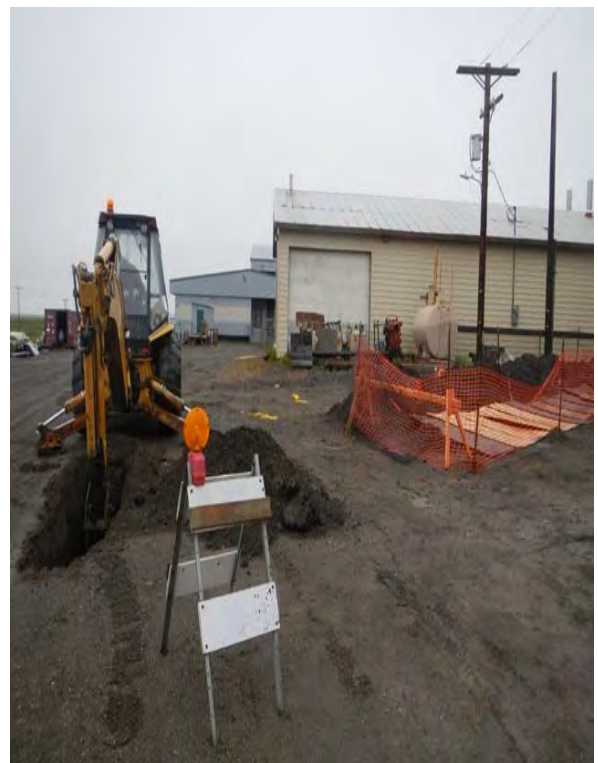
Photograph 4. Excavating Test Pit #1 (Sample Location #16). Looking toward Warm Storage Building.
