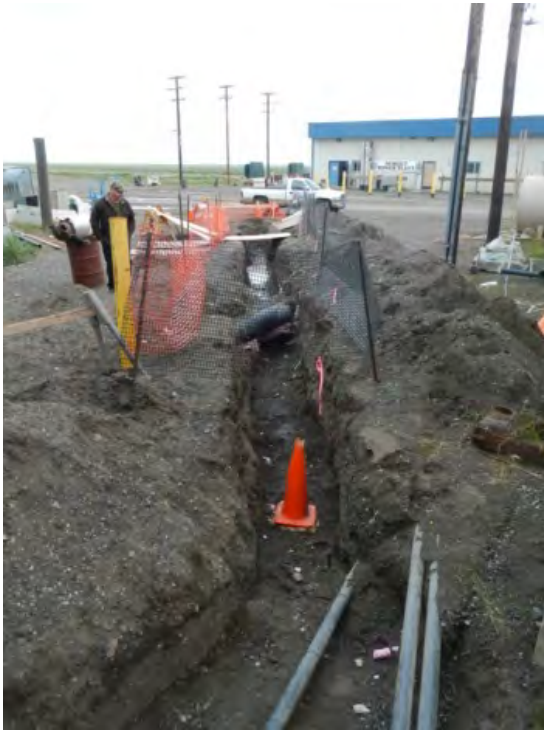
Photograph 1. Trench A looking toward Nuiqsut Power Plant Building.
