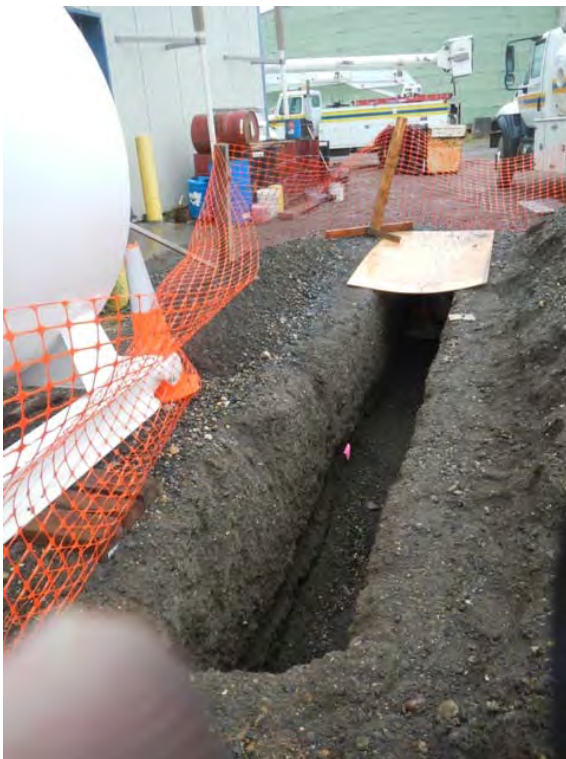
Photograph 3. Trench B looking toward Warm Storage Building.
