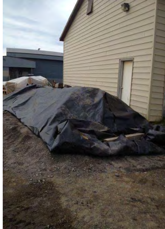
Photograph 6. Stockpile of soil exceeding 20 ppm on PID. Looking toward the school.
