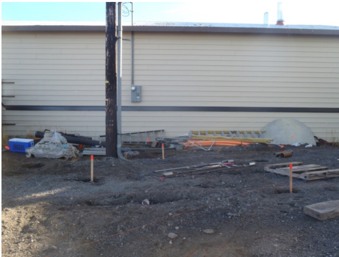
4) Locations of borings SB-01, SB-09, SB-10, and SB-18, facing south.
