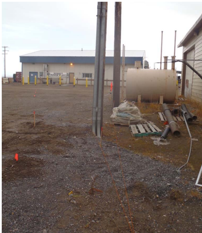
4) Borings and estimated locations of underground utilities in area, facing west.
