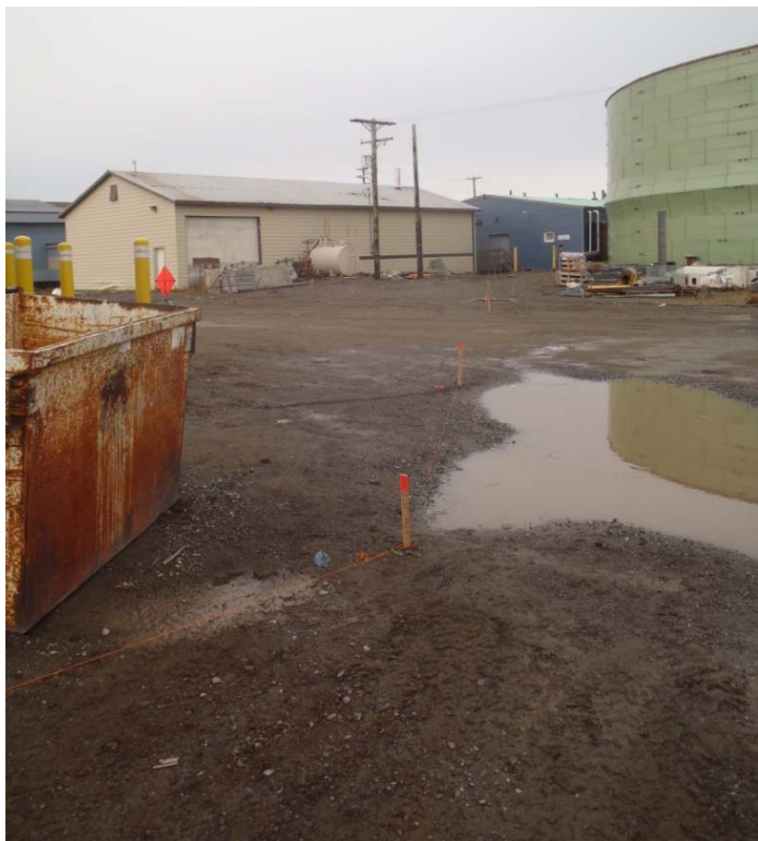
1) Estimated location of fuel line installed in 2012 (marked with lath and string), facing southwest.
