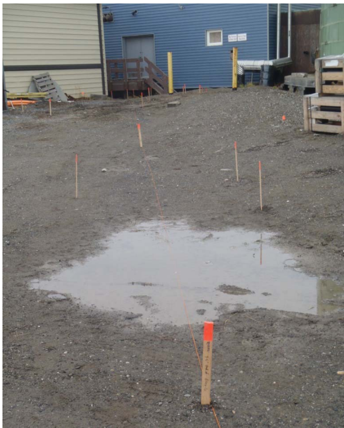
2) Estimated location of fuel line installed in 2012 (marked with lath and string), facing southwest.
