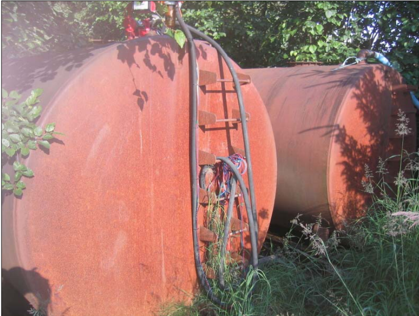
PHOTO 11 10,000 Gal. AST's at Area B looking looking east.
