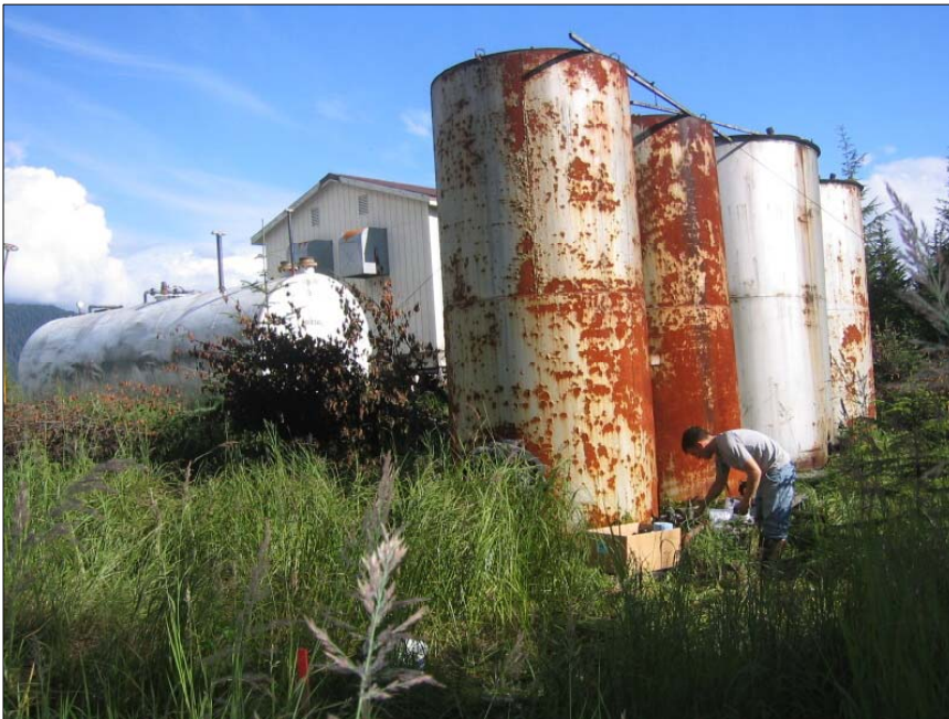
PHOTO 2 Old Tanks at Area A looking southeast. New 10,000 Gal AST and generator building in background.
