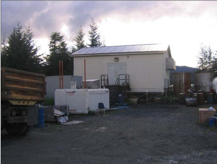
PHOTO 5 New generator building looking west. Note 2,000 Gal. vaulted AST in foreground.
