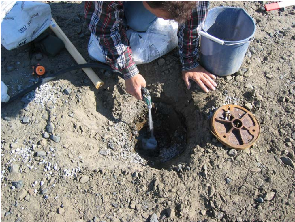
MW-3 Being Filled with 3/8-inch Bentonite Chips and Saturated with Water
