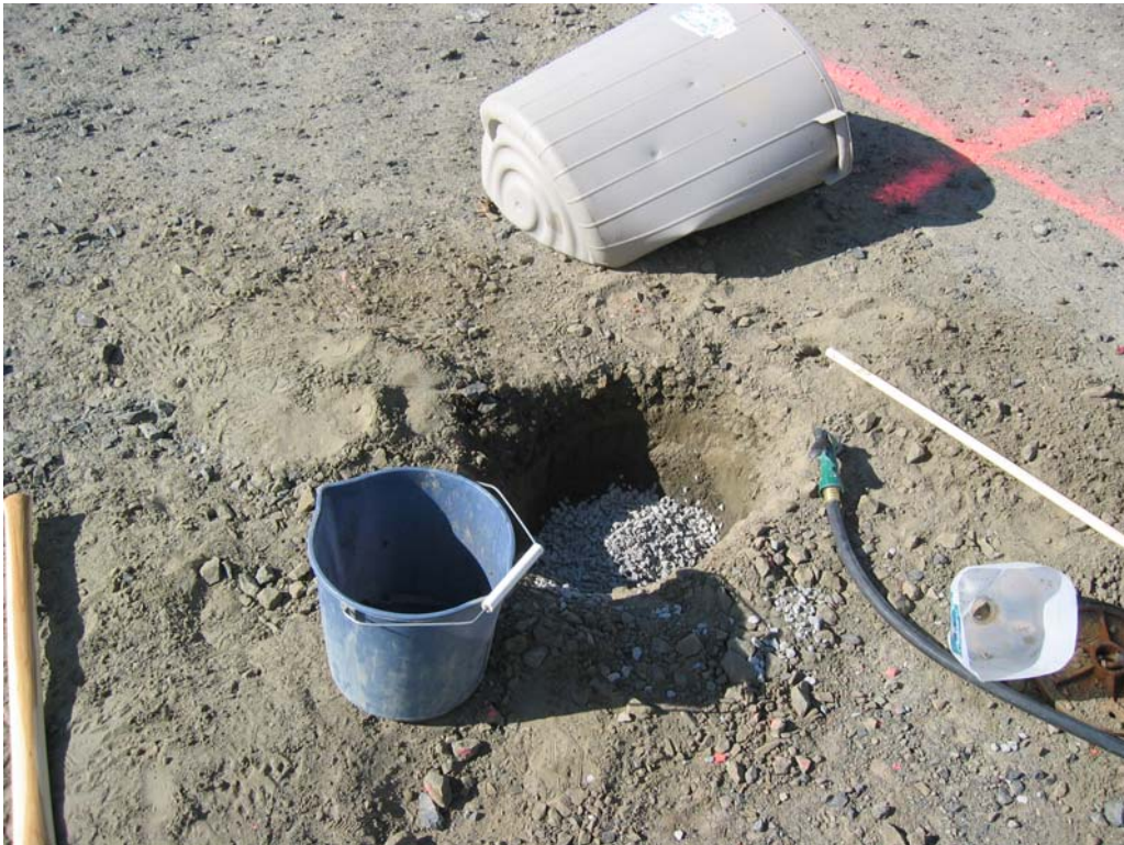
Excavated Area Backfilled with 3/8-inch Bentonite Chips (MW-4)
