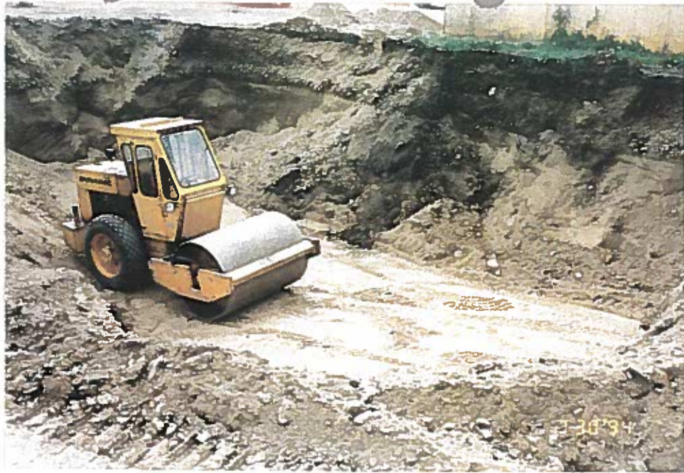
Photo 31: View of tank area during backfill and compaction.
