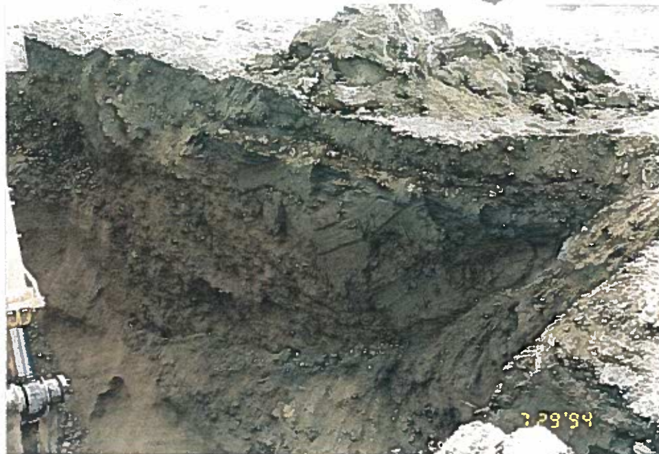
Photo 29: View of tank area south sidewall during contaminant tracking. Note highly variable conditions.
