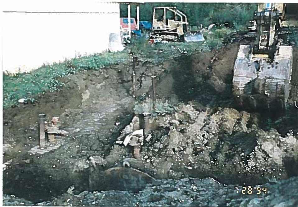
Photo 14: Excavation in tank area, exposing tank tops.
