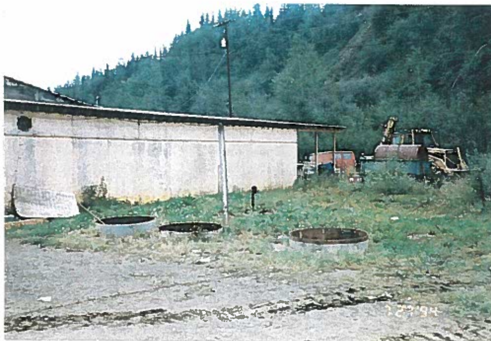
Photo 2: Tank area before excavation.
