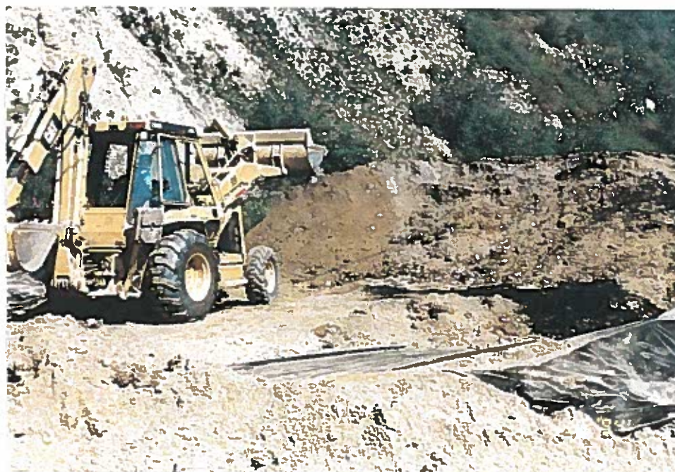
Photo 30: Formation of impacted soil stockpile.
