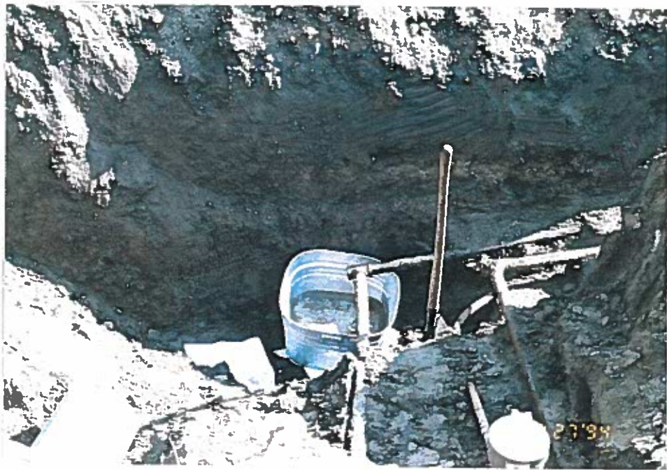
Photo 12: All lines were drained prior to cutting and removal.
