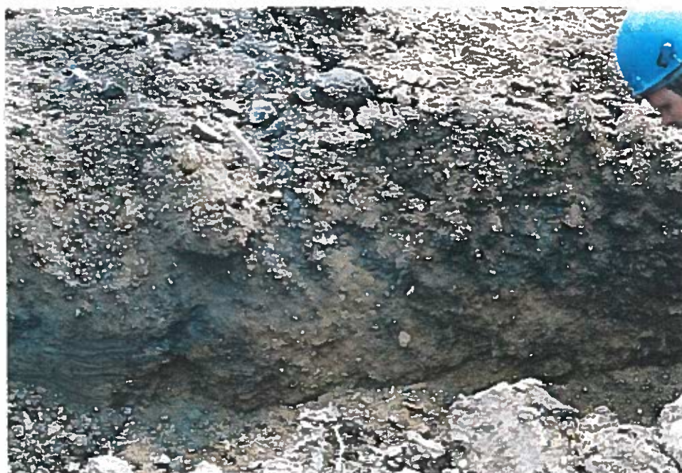
Photo 8: Grey staining was evident at the location of the tank fill piping.
