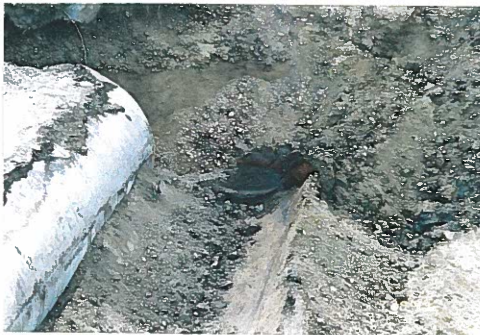
Photo 20: Excavation bottom, directly beneath Tank No. 2.
