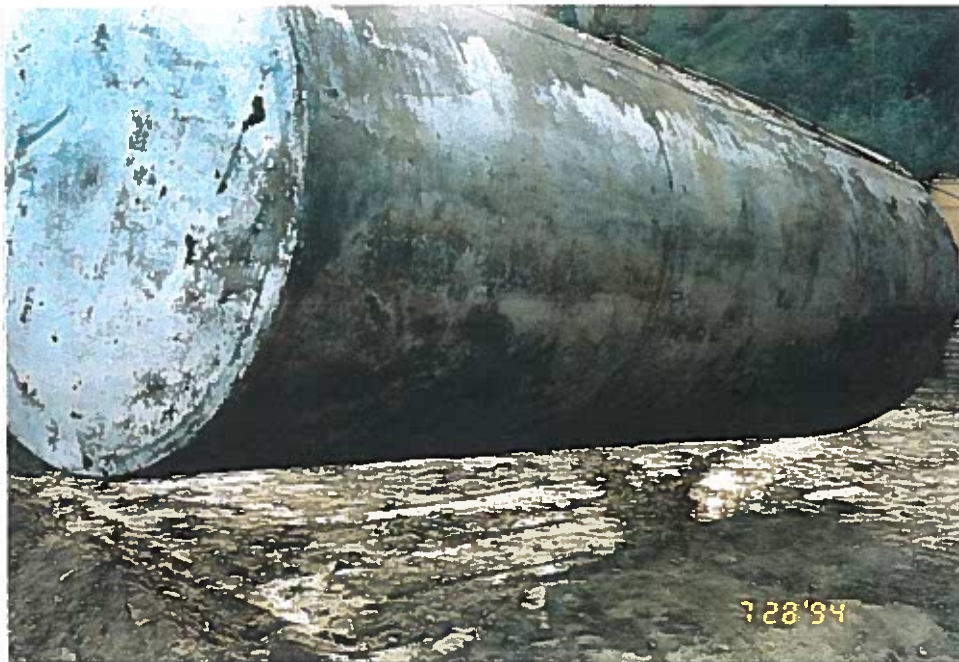
Photo 24: Close-up view of the bottom of Tank No. 3.
