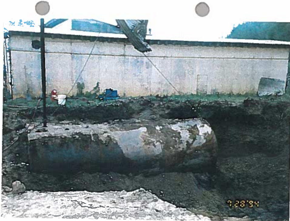
Photo 19: Removal of 4,000-gallon tank (Tank No. 2).
