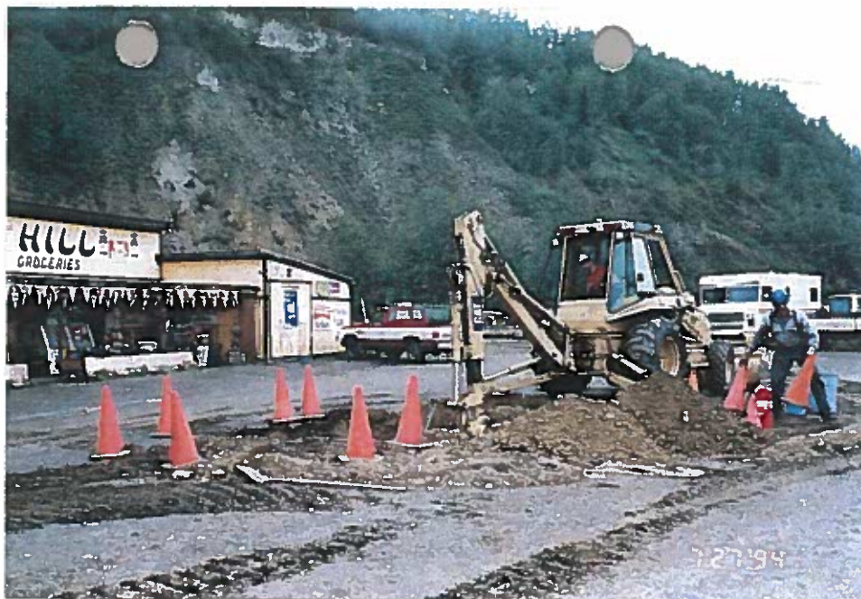
Photo 7: Site work in dispenser island area.
