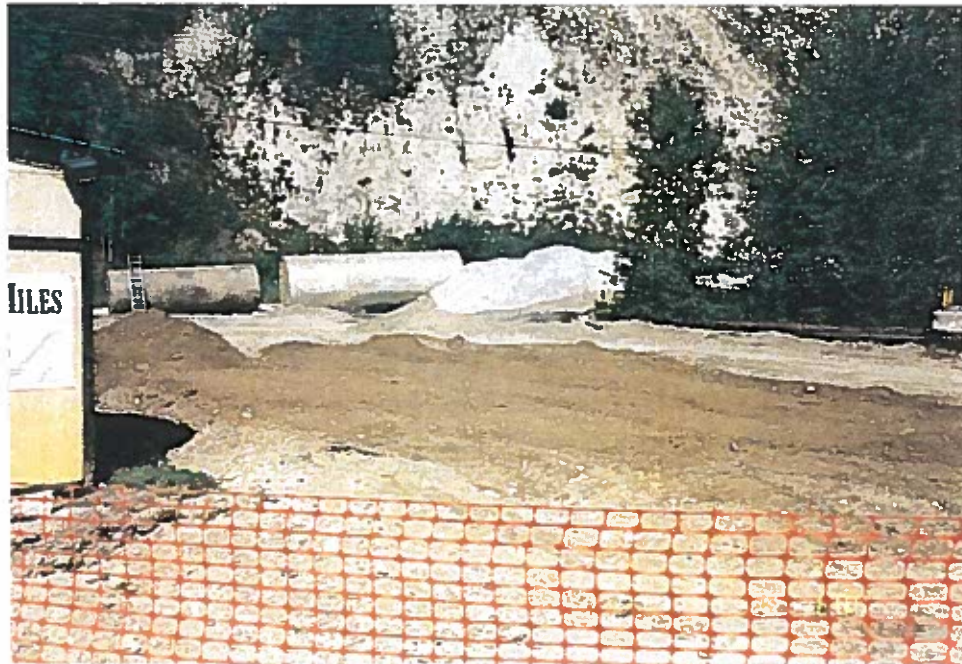
Photo 32: View of site during final grading.
