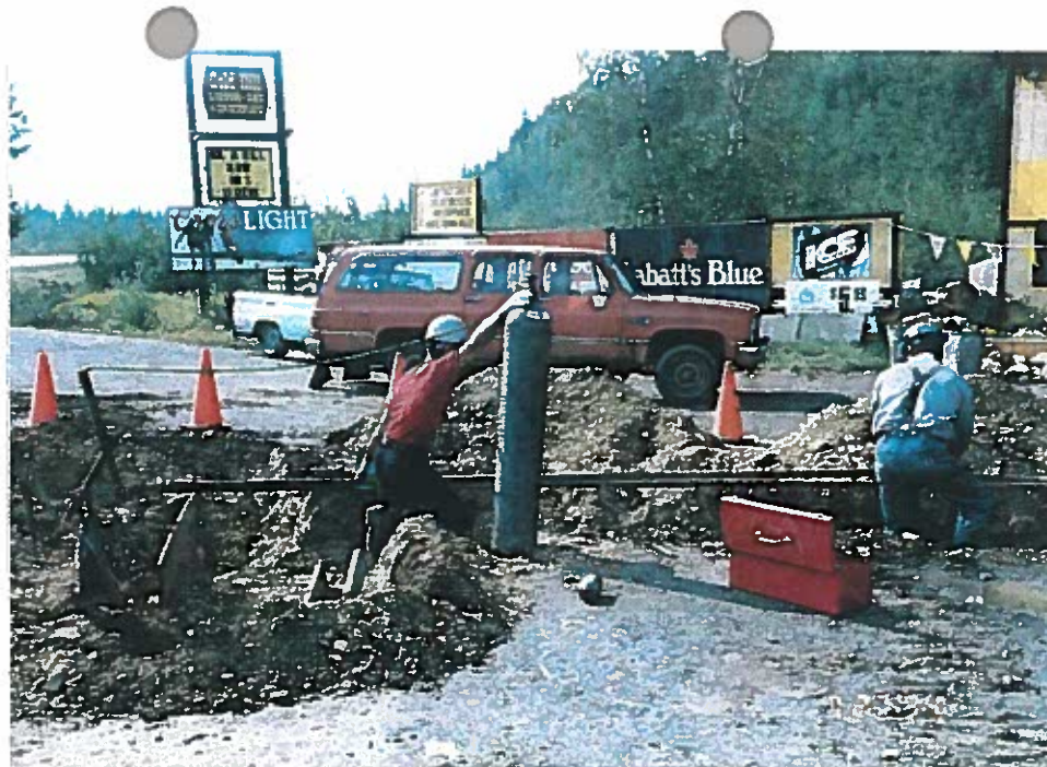
Photo 13: Lines were purged with CO 2 prior to and during pipe cutting.
