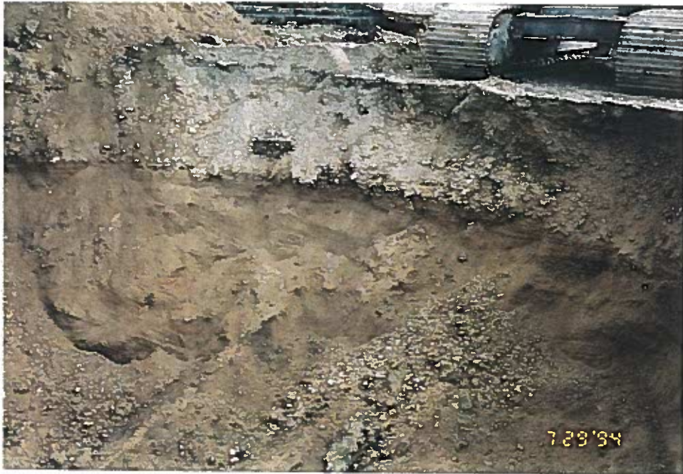
Photo 26: Soil conditions along the eastern sidewall of the tank excavation area.
