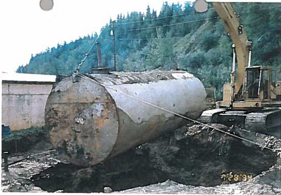
Photo 17: Removal of 10,000-gallon tank (Tank No. 1).
