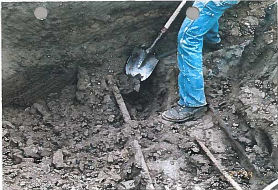
Photo 11: Hand-digging near fuel lines. Note wood support at photo center.
