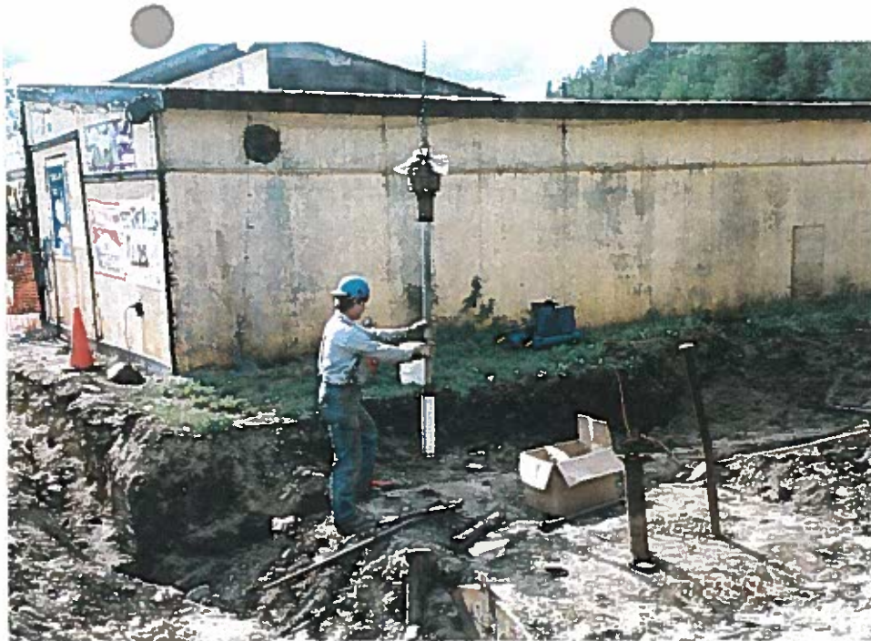
Photo 15: Removal of turbine pumps.
