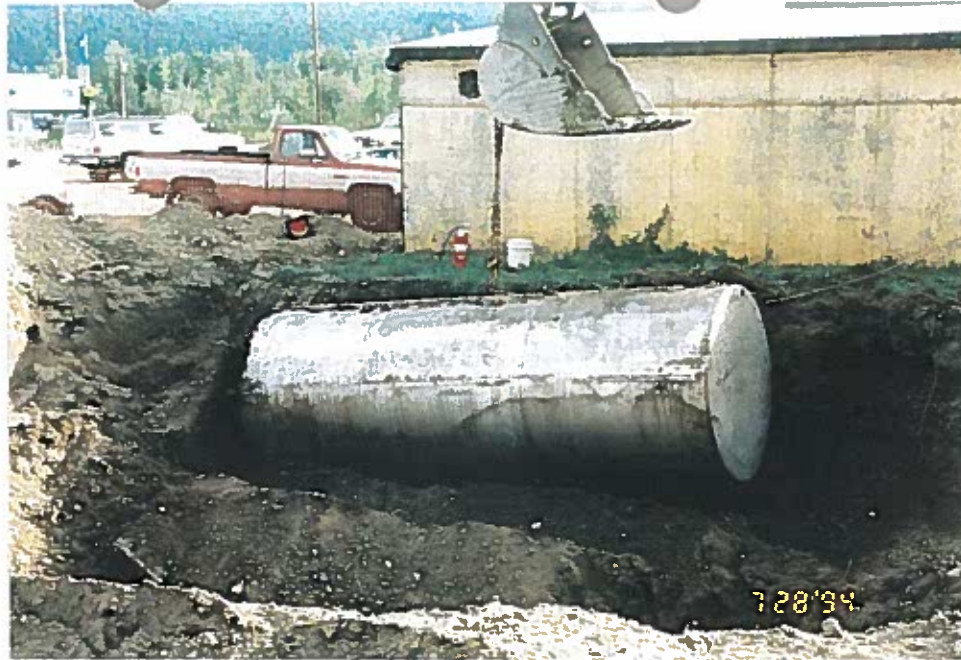
Photo 23: Removal of Tank No. 3.
