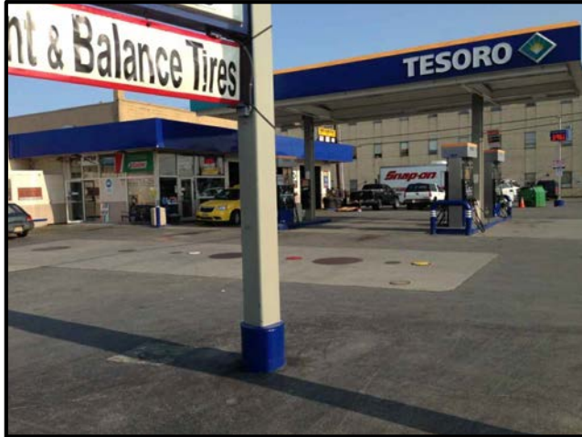
1. View of Site facing North
