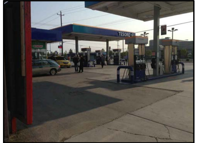
2. View of Site facing Northeast
