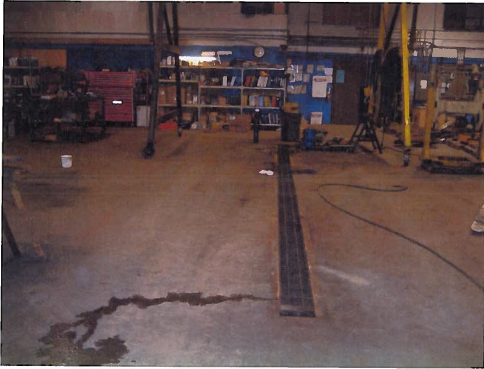
Photo 01 - Trench drain in main shop floor as originally constructed
