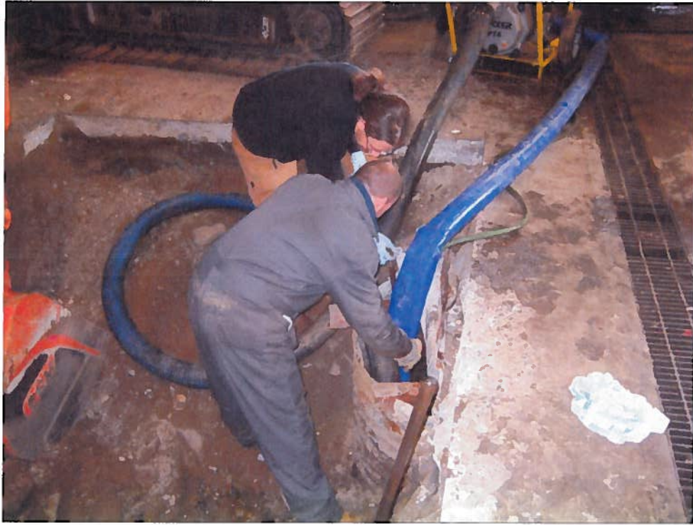
Photo 03 - Removal of liquid and sludge from former dry well structure
