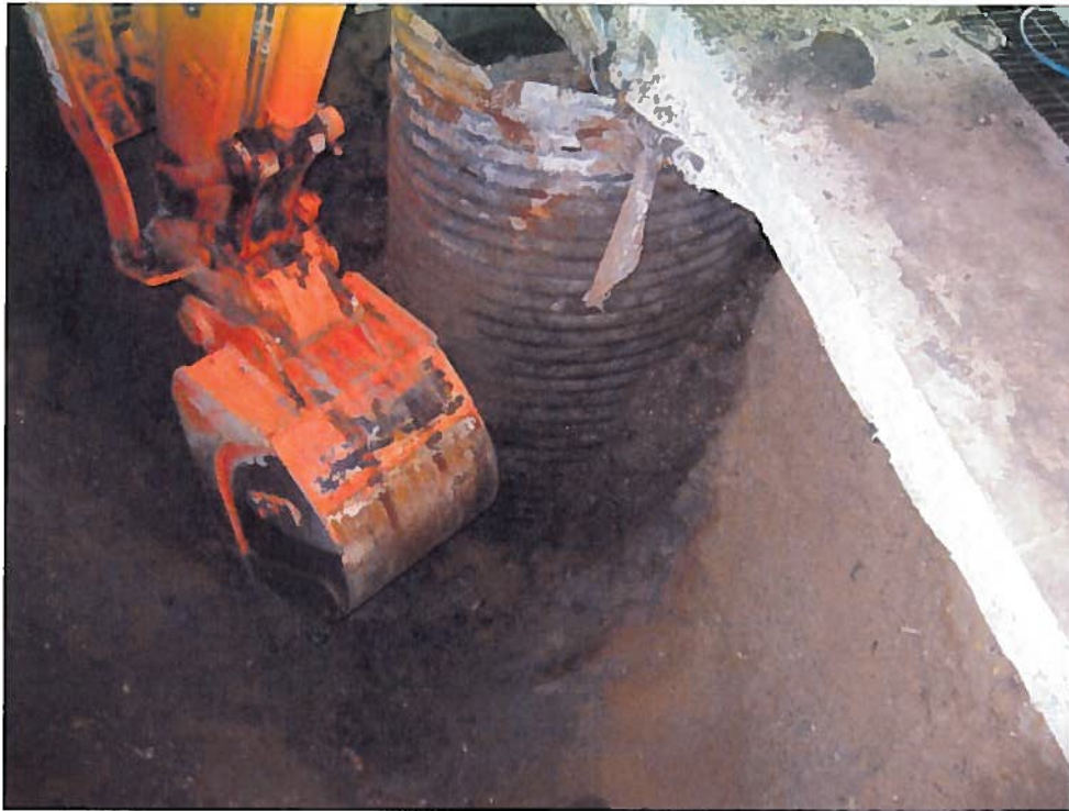
Photo 04 - Excavation of contaminated soil adjacent to former dry well structure
