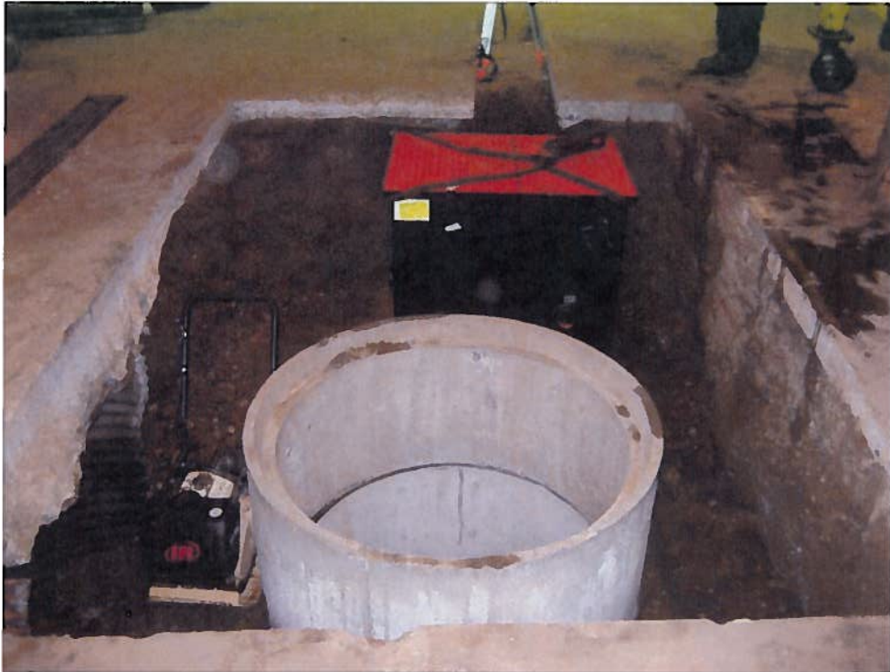
Photo 08 - During installation of oil water separator system (sediment trap in foreground)
