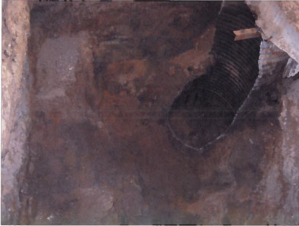
Photo 07 - Final limits of excavation prior to oil water separator system installation
