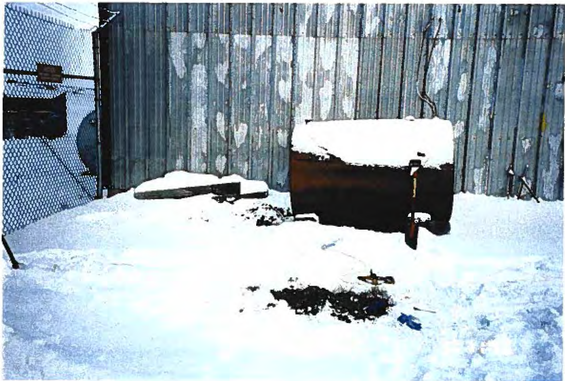
500-Gallon Heating Oil AST and Sample Location 96-N-02 (Looking West), 10-11-96
