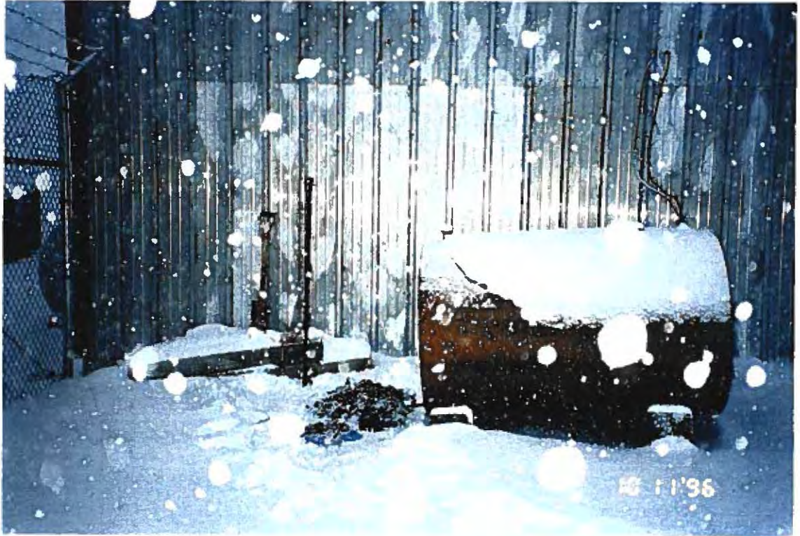
500-Gallon Heating Oil AST and Sample Location 96-N-01 (Looking West), 10-11-96
