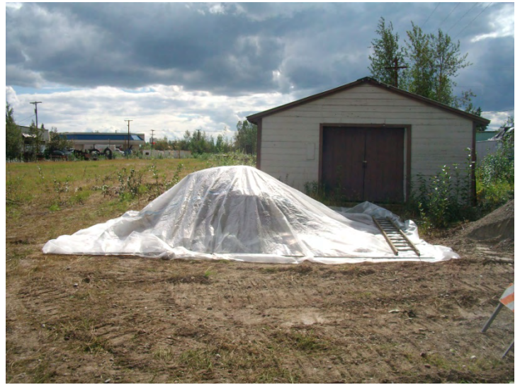
Photo 20. Stockpiled Soils From Septic Tank Area
