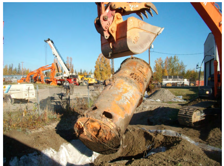
Photo 24. Removal of the Septic Tank
