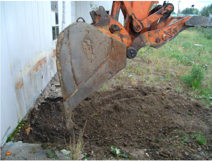
Photo 1. Former Used-Oil AST Excavation
