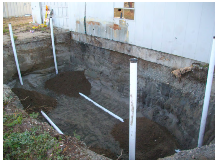
Photo 6. Drain Tile & Solid Risers in Former Used-Oil Excavation
