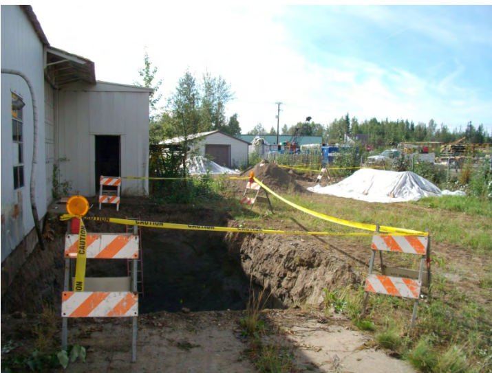
Photo 5. Barricaded Former Used-Oil AST Excavation
