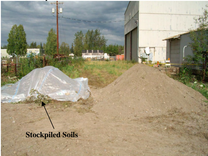
Photo 21. Stockpiled Soils From Septic Tank Area
