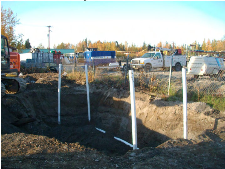
Photo 15. Drain Tile & Solid Risers in Fuel Line Excavation
