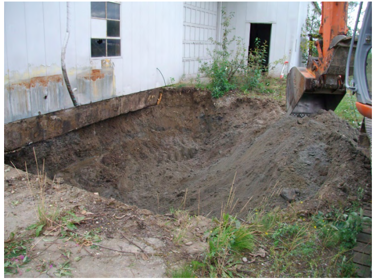
Photo 2. Former Used-Oil AST Excavation
