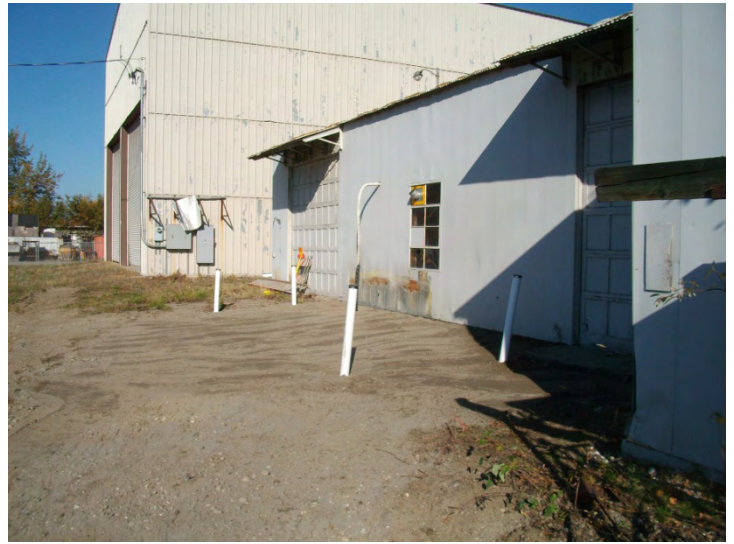
Photo 8. Former Used-Oil AST Excavation
