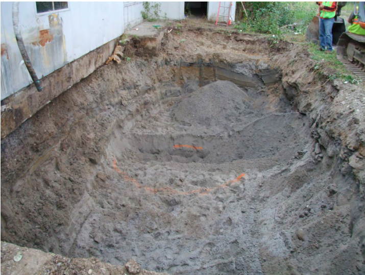
Photo 3. Former Used-Oil AST Excavation
