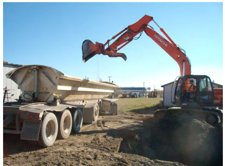
Photo 12. Former Septic Tank Excavation
