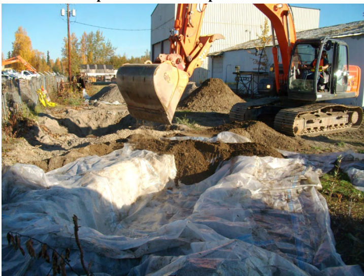
Photo 23. Shallow Containment Trench for Sludge
