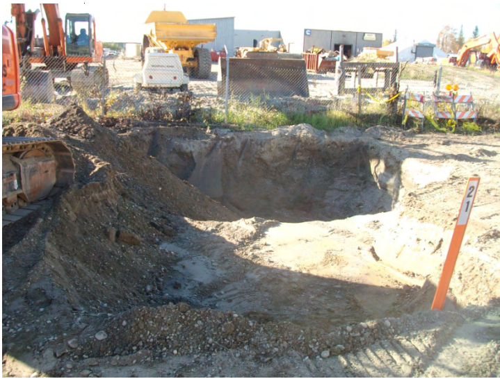
Photo 13. Fuel Delivery Line Excavation
