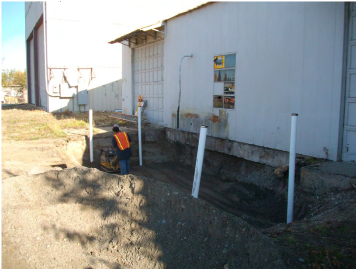
Photo 7. Compaction of Former Used-Oil AST Excavation
