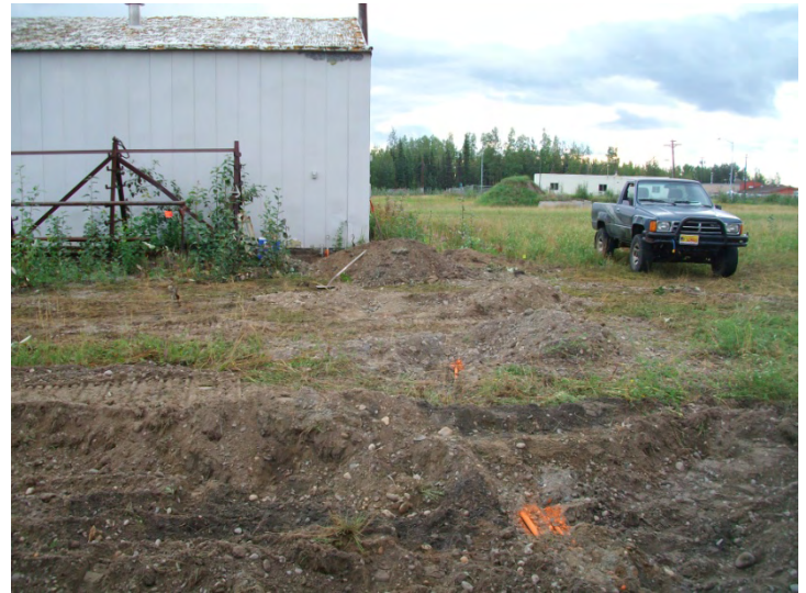
Photo 10. Fuel Delivery Line
