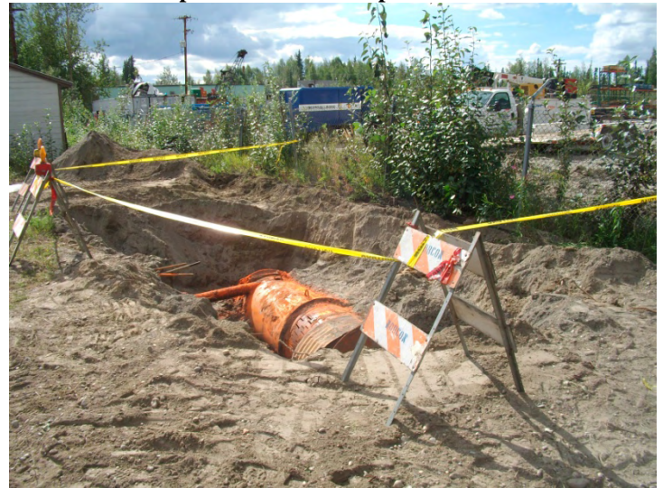
Photo 22. Barricaded Septic Tank Excavation
