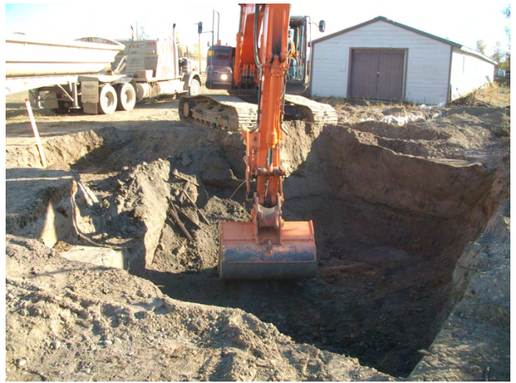
Photo 14. Fuel Delivery Line Excavation
