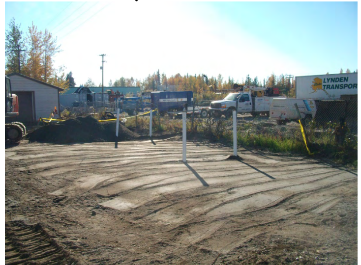
Photo 16. Backfilled Fuel Delivery Line Excavation
