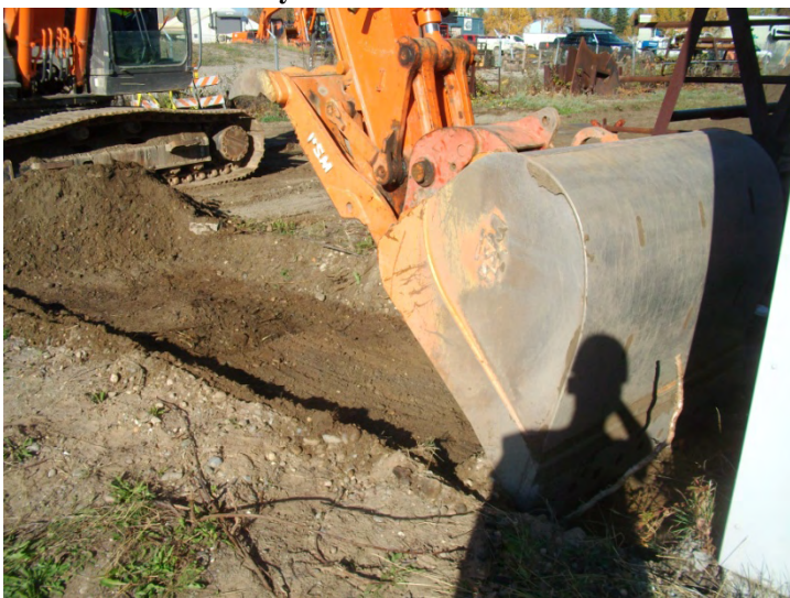
Photo 11. Fuel Delivery Line Excavation
