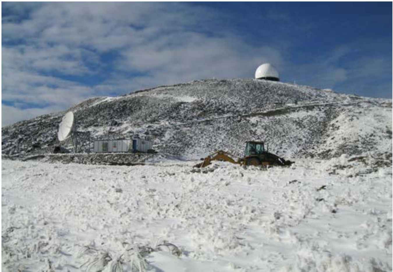
Test pit excavation at the WACS (2011)
