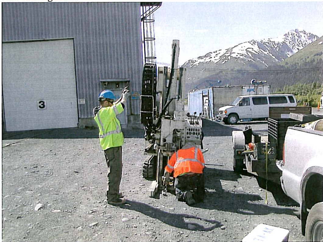
Photograph 2: Purging and sampling temporary monitoring well MW-1. View to the south.
