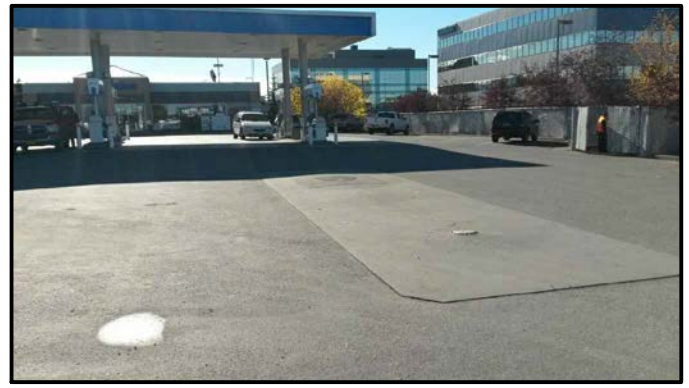
Photo 4. View of site looking south from the north end of the site
