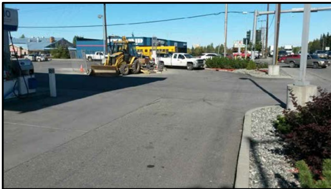
Photo 3. View of site looking north from the east side of the site
