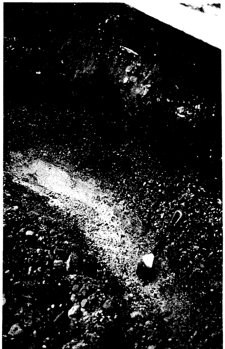
PHOTO 6 - DEG Excavation- Yard Fill Overlying DEG Gravel Pad w/ Lube Oil Overlying Sandstone Bedrock (minimal penetration)
