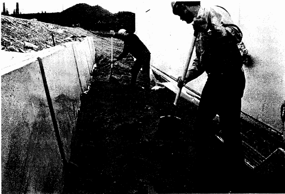
PHOTO 7 - DEG Source Area Backfill, Liner Placement and Grading
