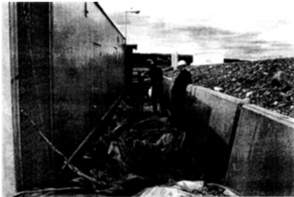
PHOTO 4 - Well Point Installation in Lube Oil Spill Source Area at the DEG
