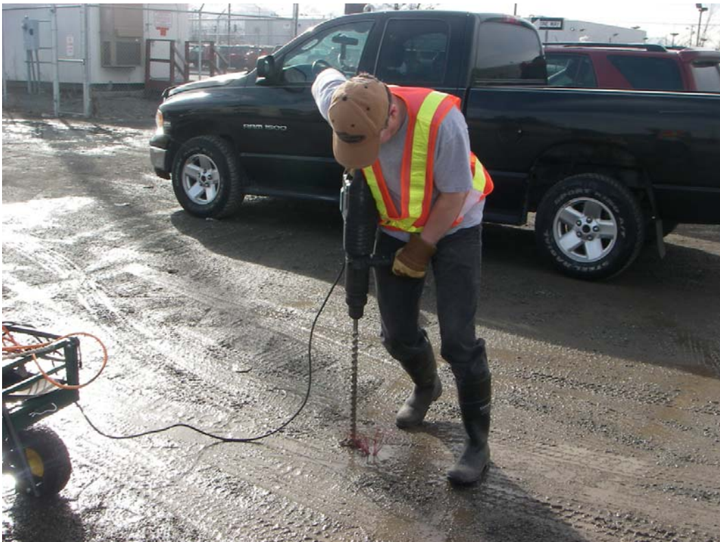
Photograph 4. Drilling passive soil gas monitoring points in April.
