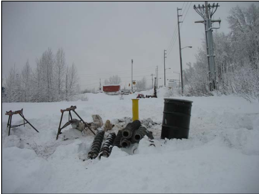
Time: 2:10 Date: 1/11/07 Direction: South Description: BH-1; MW-1 well stand in center.
