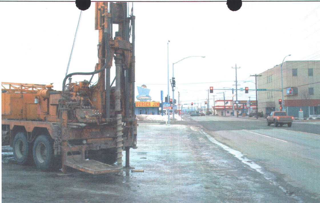
Photo 1. Advancing Boring MW-2 (looking south)
