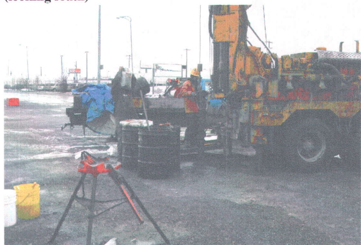
Photo 3. Advancing Boring MW-4 (looking southeast)
