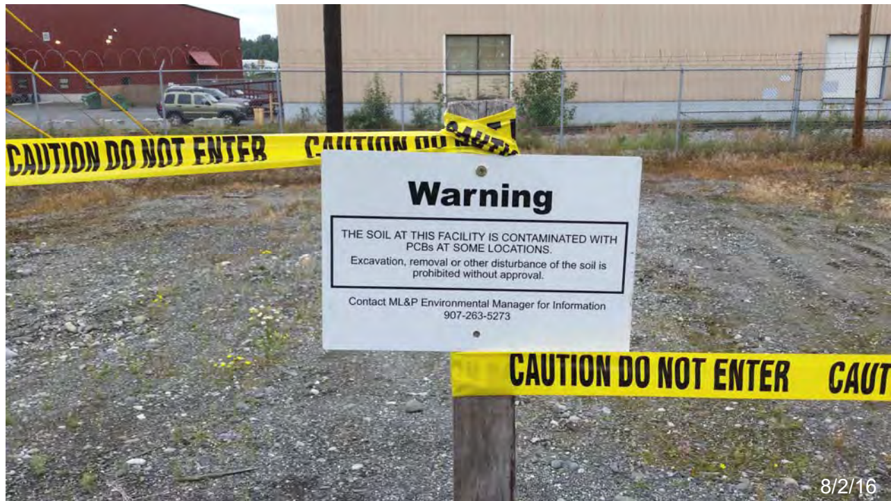
Photo 14. Signs were posted on the cordoned off area to alert site workers and direct questions to the ML&P Environmental Manager.
