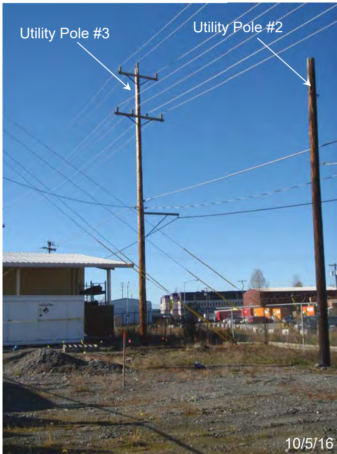
Photo 5. Composite sampling in the central portion of the project area, during the October sampling event. Utility poles #2 and #3 are indicated. Utility pole #3 is located within composite sample AP-32 (PCB = 89.4 mg/kg) and will need to be stabilized during contaminated soil excavation. Photo faces west.
