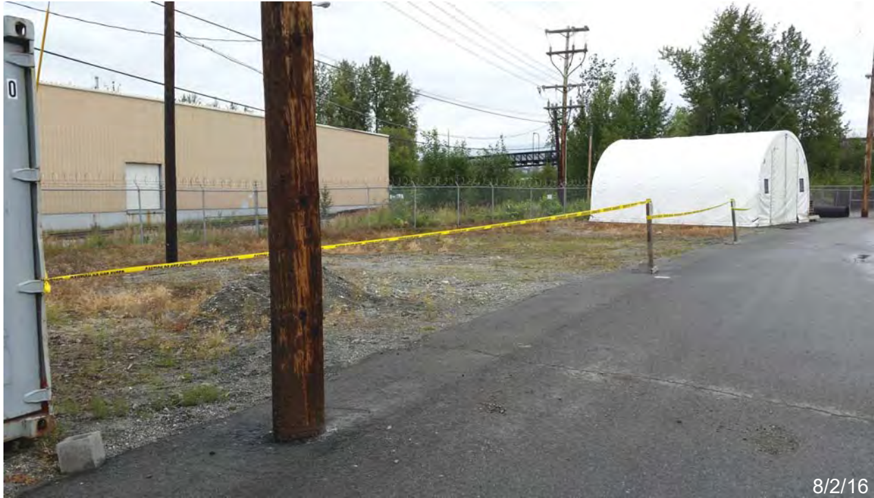
Photo 13. Following receipt of June 2016 sample results, ML&P cordoned off the unpaved area where soil contains PCBs >50 mg/kg. Photo faces northeast.
