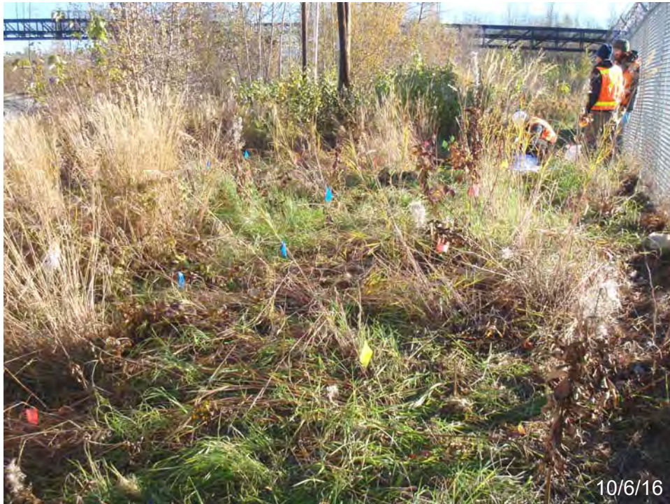
Photo 16. Layout of the sample grid north of the facility fence and collection of soil samples. Samples NF-12 and NF-13 are in the foreground. The entire area was vegetated, requiring removal of grass and roots prior to collection of underlying mineral soil. Photo faces east.
