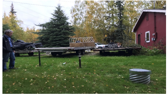
Photo 4: Underground storage tank and culvert (Facing north)
