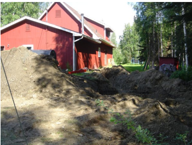
Photo 3: Site Excavation photo (Facing east, predating 2018)
