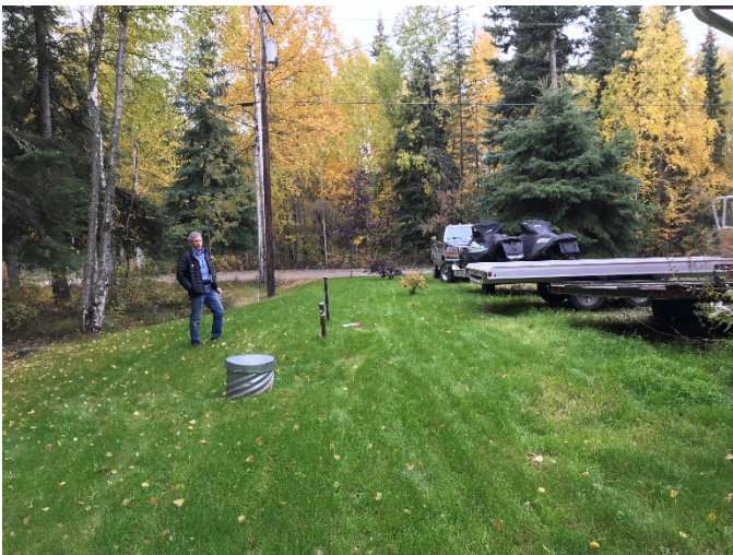
Photo 2: Underground storage tank and culvert (Facing west)
