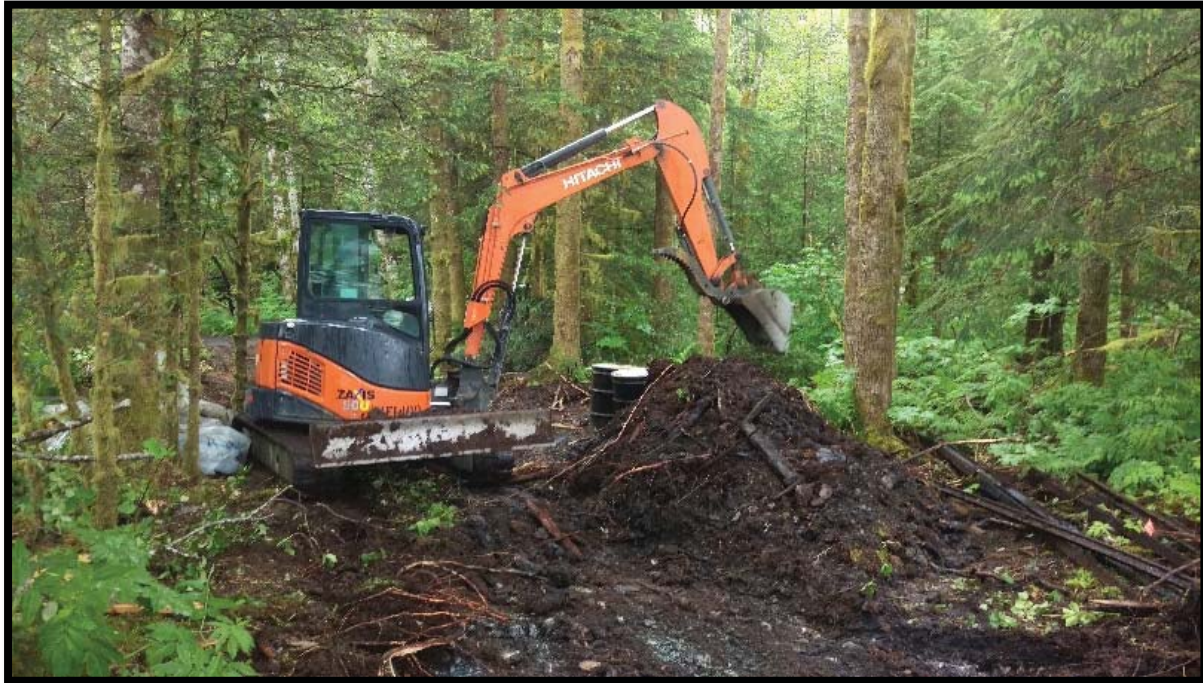
Photo 3: Stockpiling the soil before removal from the site.
