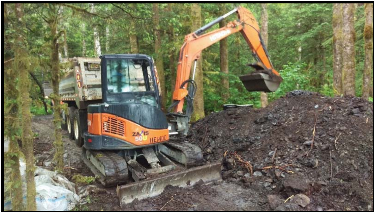
Photo 8: One of five dump truck loads of soils removed and transported to Bicknell landfarm.
