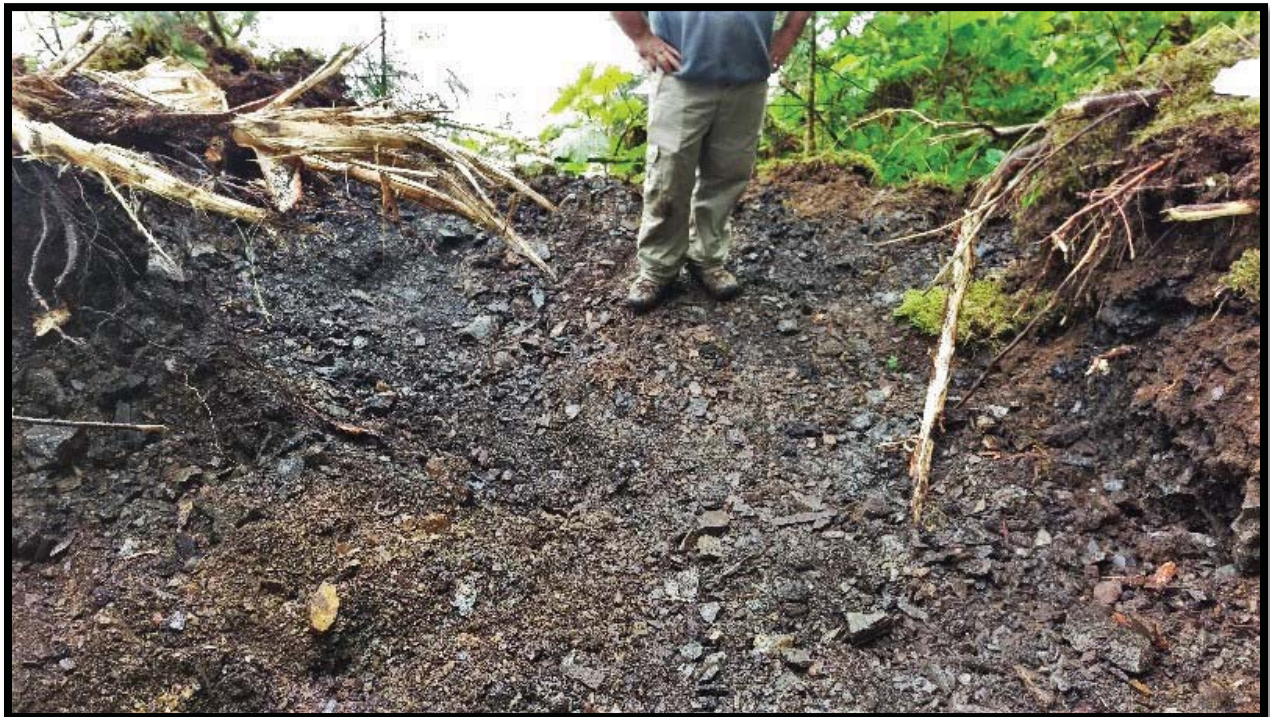
Photo 6: The entire north east bank was completely removed to a depth of approximately 2.5 – 3 ft.
