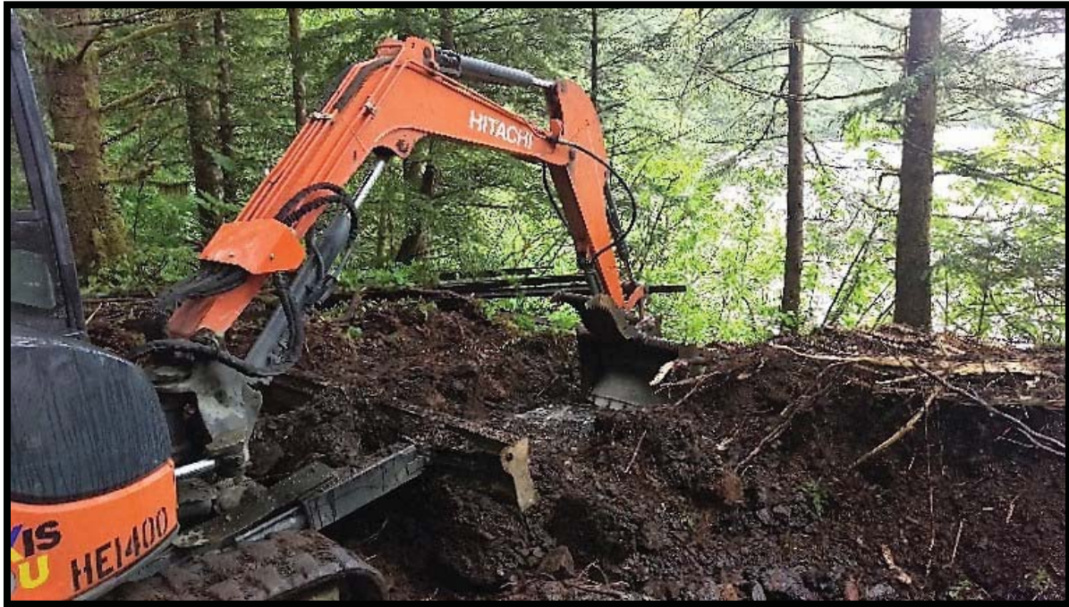
Photo 7: View of northwest cut. Note excavator cut away to the edge.
