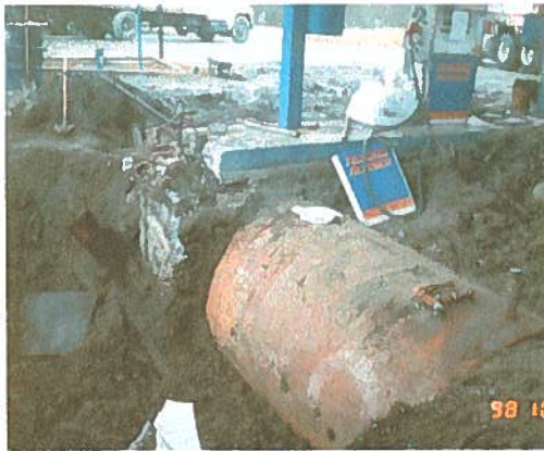
Excavation shows concrete that was poured around the 2,000 gallon UST.
