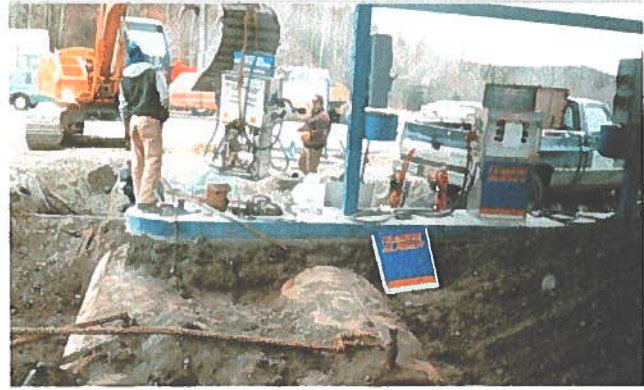
USTs as they are being uncovered.
