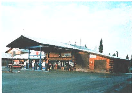
Gasoline dispenser island and canopy.
