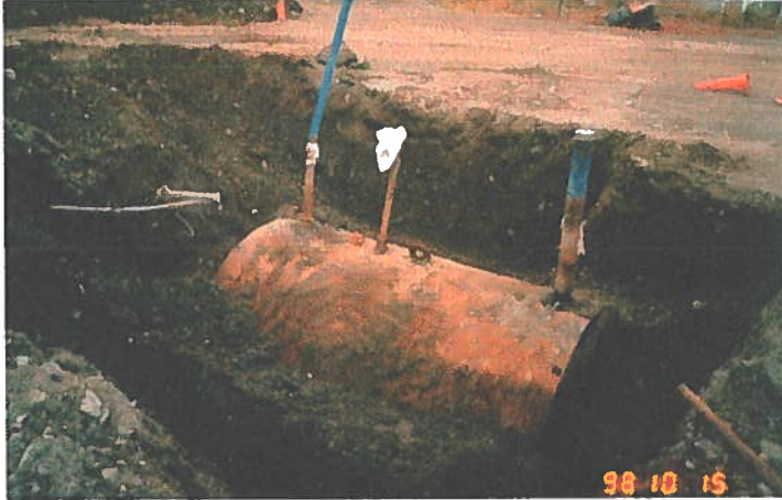
Looking north at 2,000-gallon diesel UST excavation.
