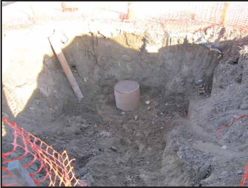
Photo 3: Typical well decommissioning, after Sonotube filled with concrete.
