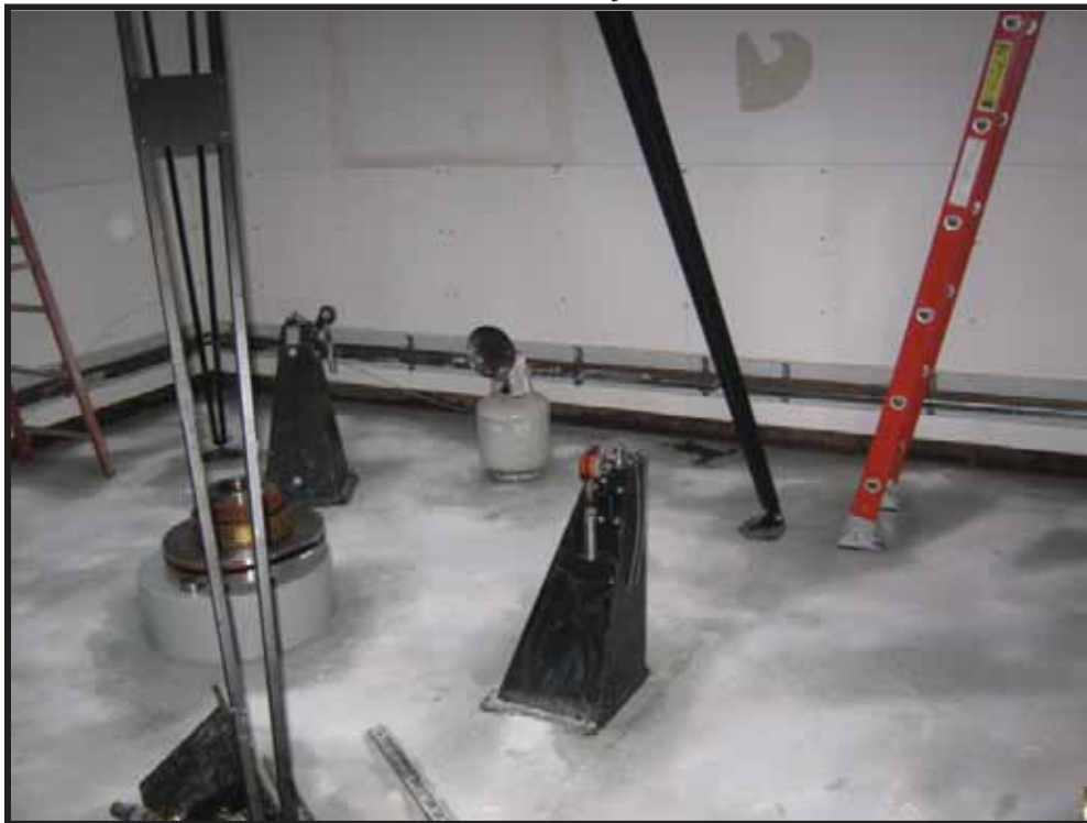
Photo 3: LMT room after removal of porous surfaces and cleaning with mercury detergent.
