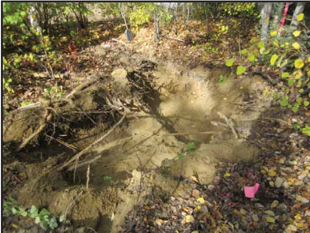
Photo 4: Final extents of excavation.
