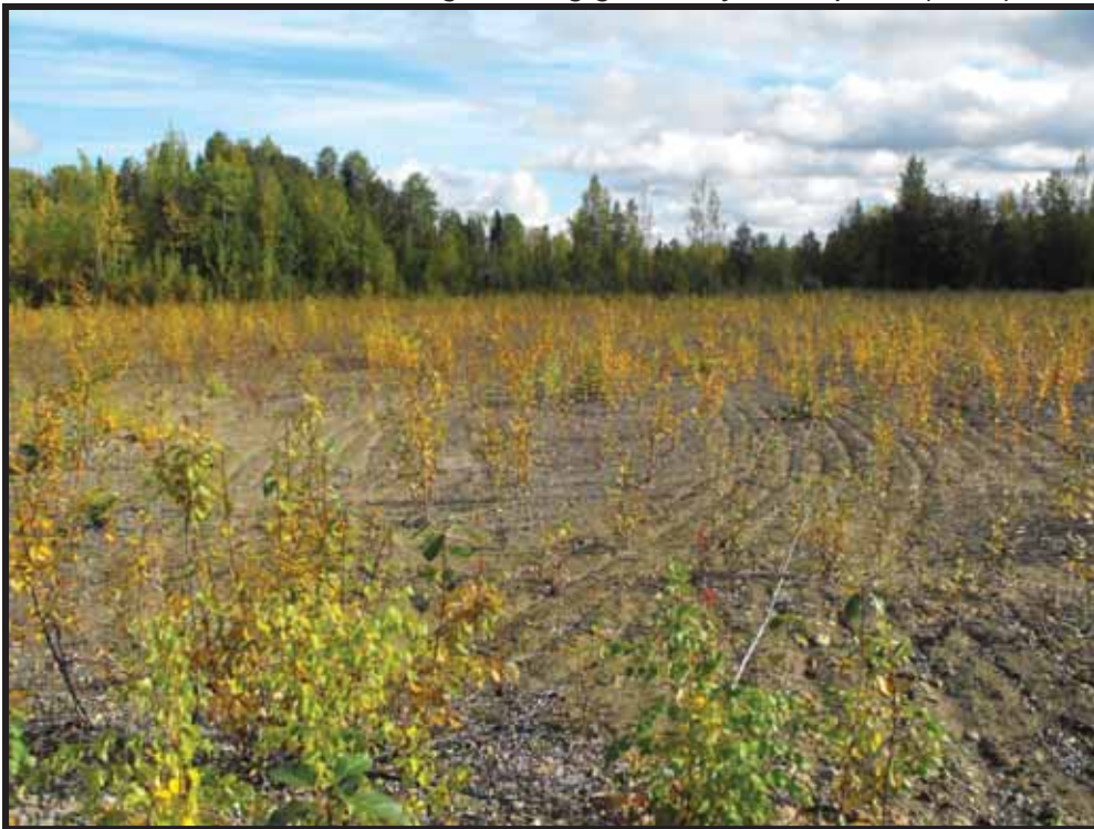
Photo 4: Looking east across Main Transmitter Array after removal and disposal of ground grid wires
