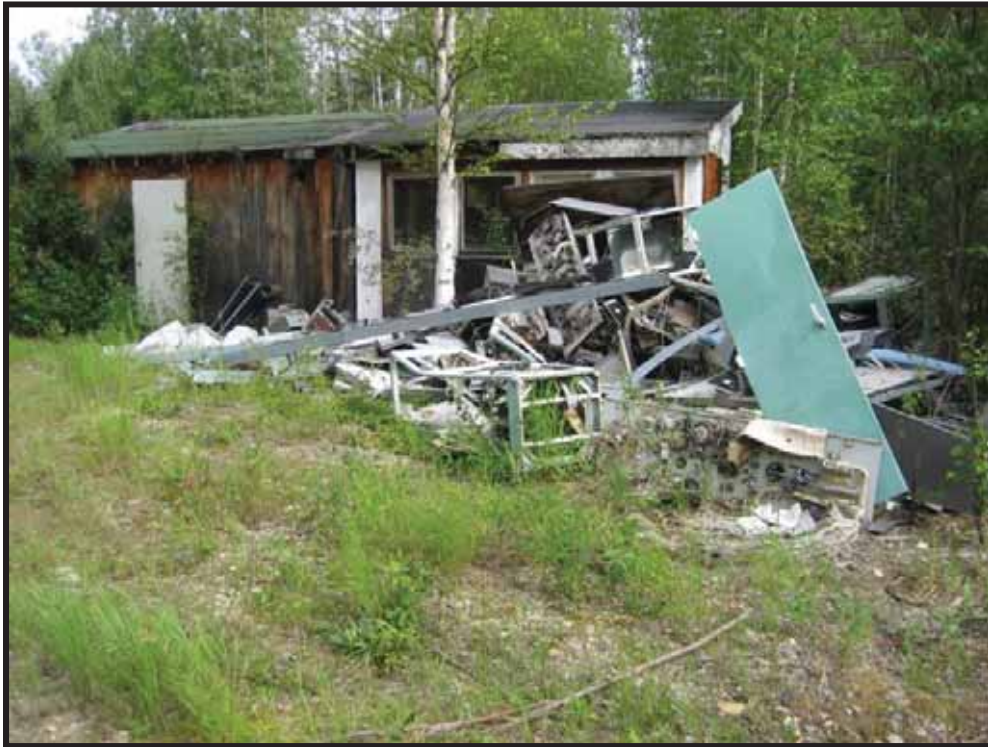
Photo 9: Looking east at debris pile and storage trailers in Boneyard area (2010)
