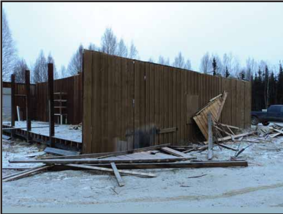
Photo 3: Photo taken facing southeast during LIDAR garage demolition.
