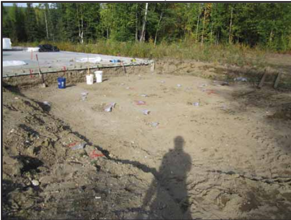
Photo 7: Final extents of excavation with field screening samples.
