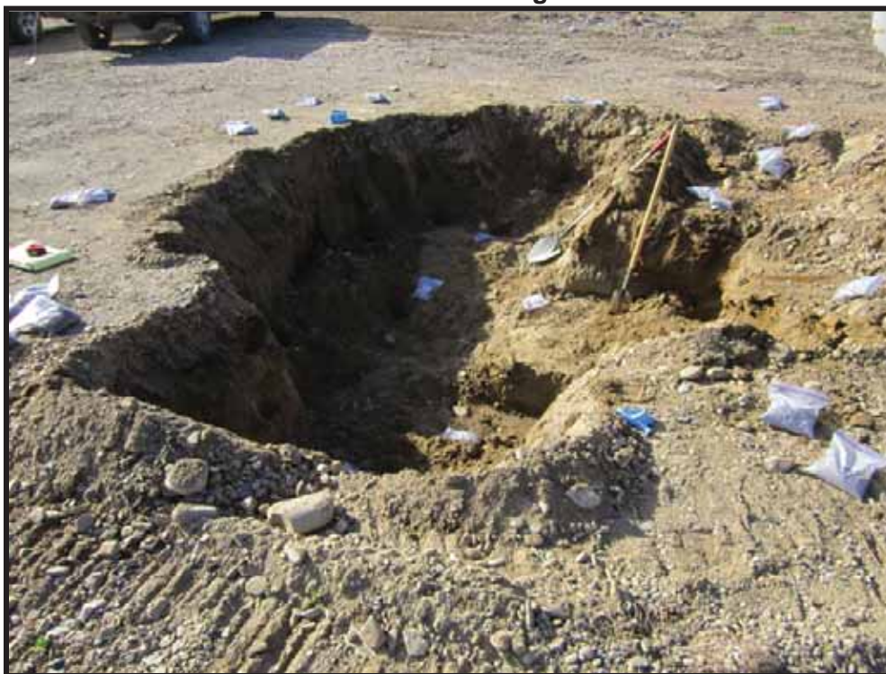
Photo 3: Looking south at final excavation limits.
