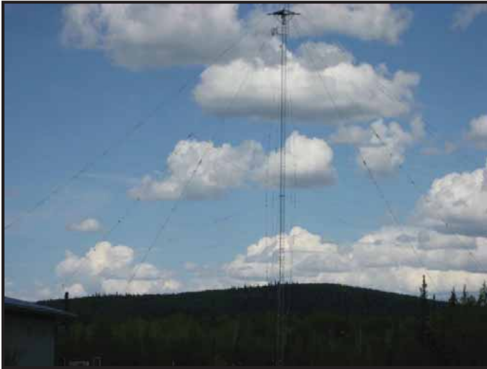
Photo 5: Looking north at square antenna field with generator building in lower left (2009)
