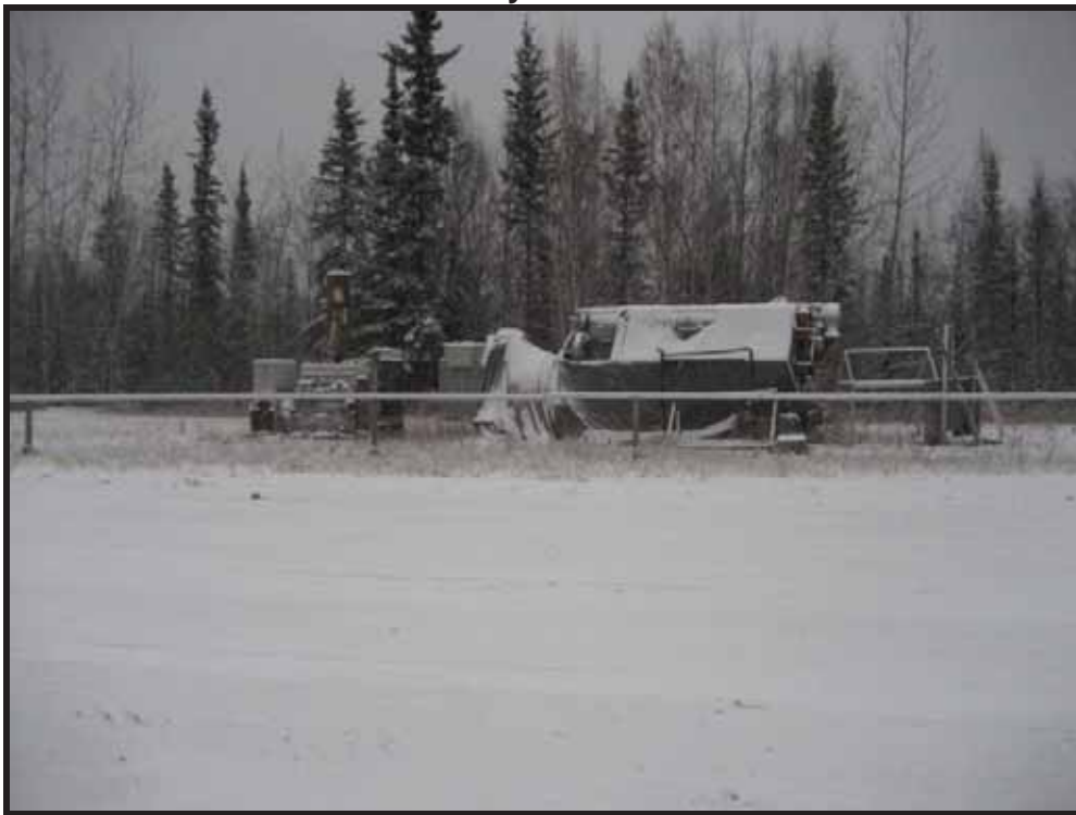
Photo 1: Looking south at the parts generator south of the powerhouse.
