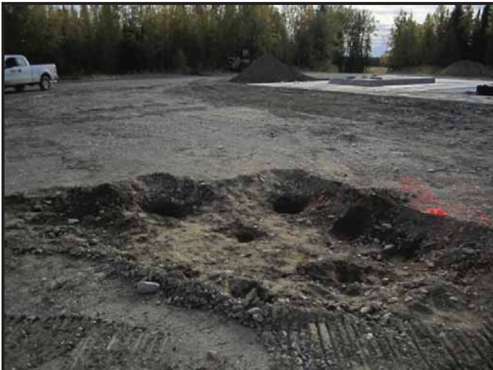
Photo 2: Photo taken facing southwest. Preliminary characterization September 2012.
