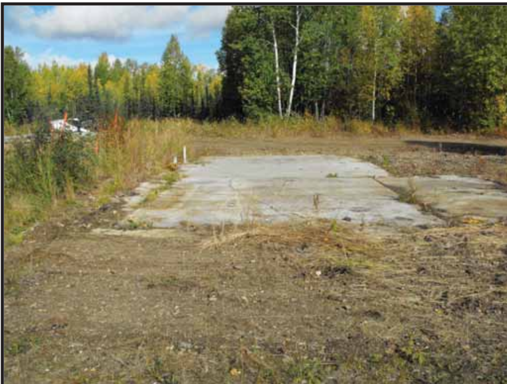
Photo 4: Photo taken facing north showing LIDAR garage slab.
