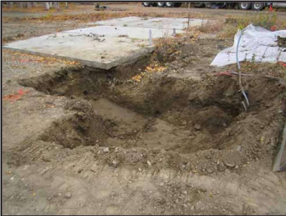
Photo 5: Photo taken facing north showing LIDAR garage soil remediation excavation.
