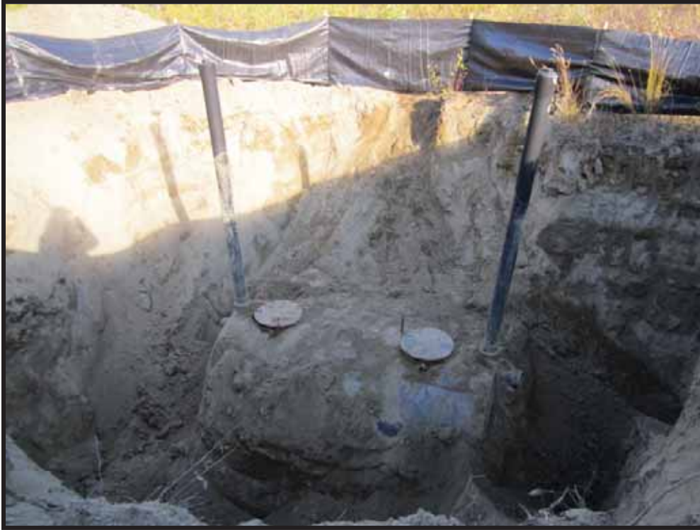
Photo 1: Typical septic tank excavation, southeast of Antenna Building.
