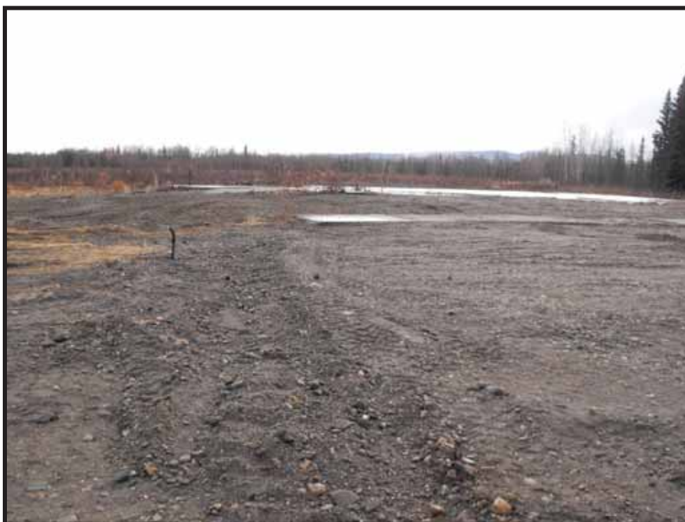
Photo 4: Excavation backfilled to grade October 2012, typical of each location.
