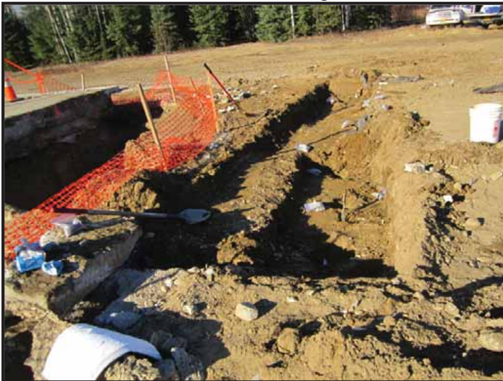
Photo 7: Excavation outside footing perimeter on east side of north pedestal.
