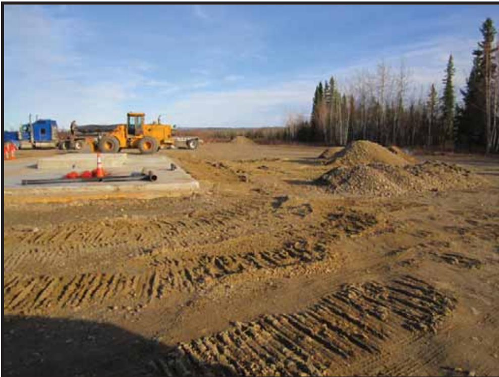
Photo 4: Typical excavation backfilled, between stockpiles of backfill material and slab.
