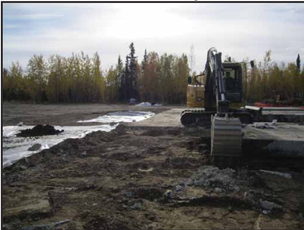
Photo 5: Excavating contaminated soils after removal of additional concrete slab.
