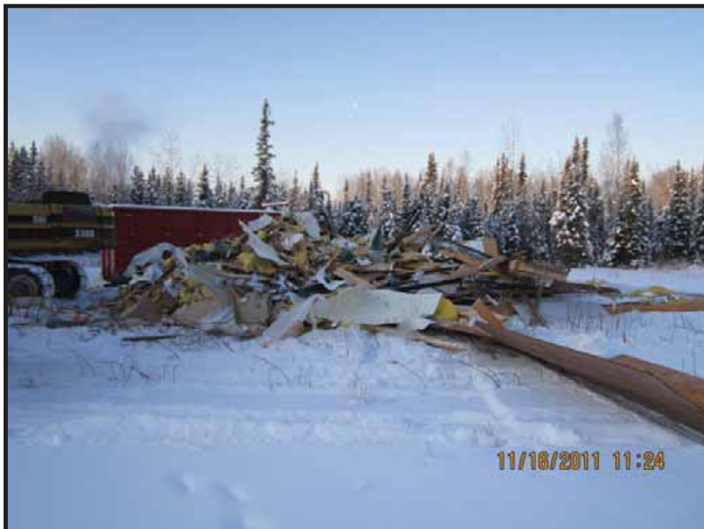
Photo 4: Building during mechanical demolition.
