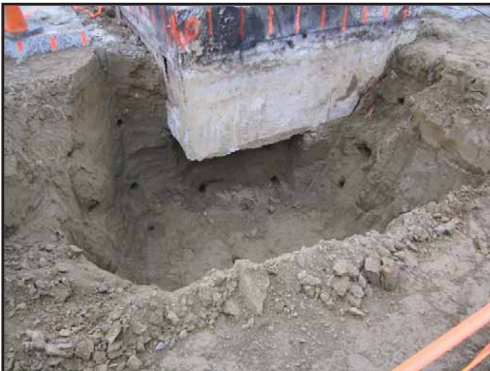
Photo 8: Final limits of excavation on east side of central pedestal. Orange markings are 1-foot demarcation lines.
