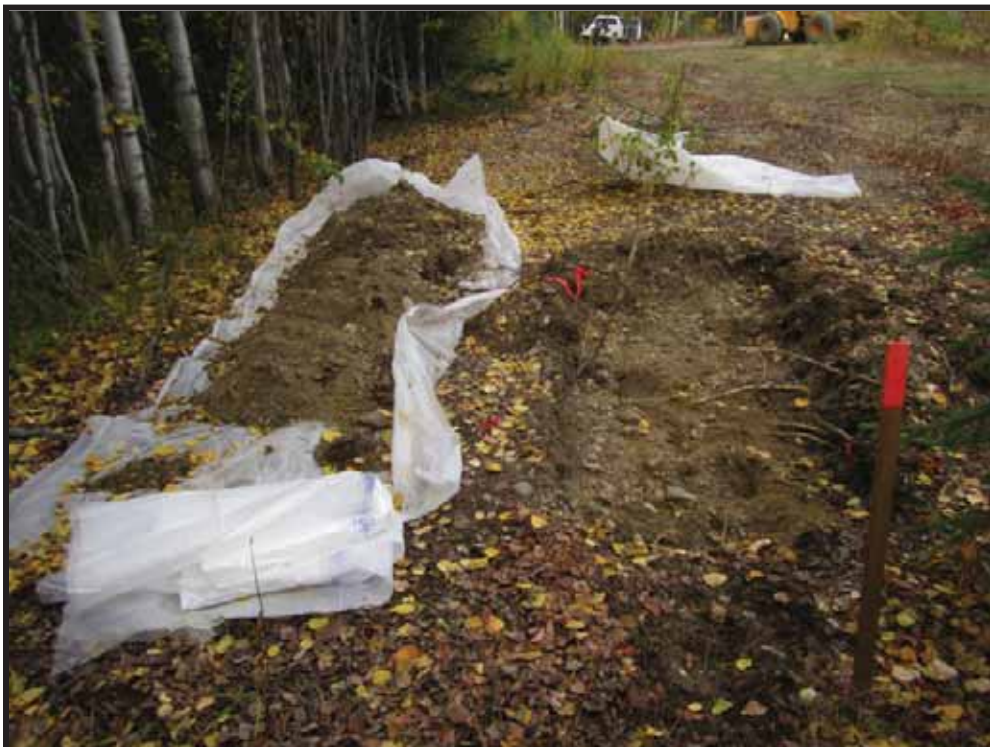
Photo 4: Final excavation limits and stockpile September 2012.
