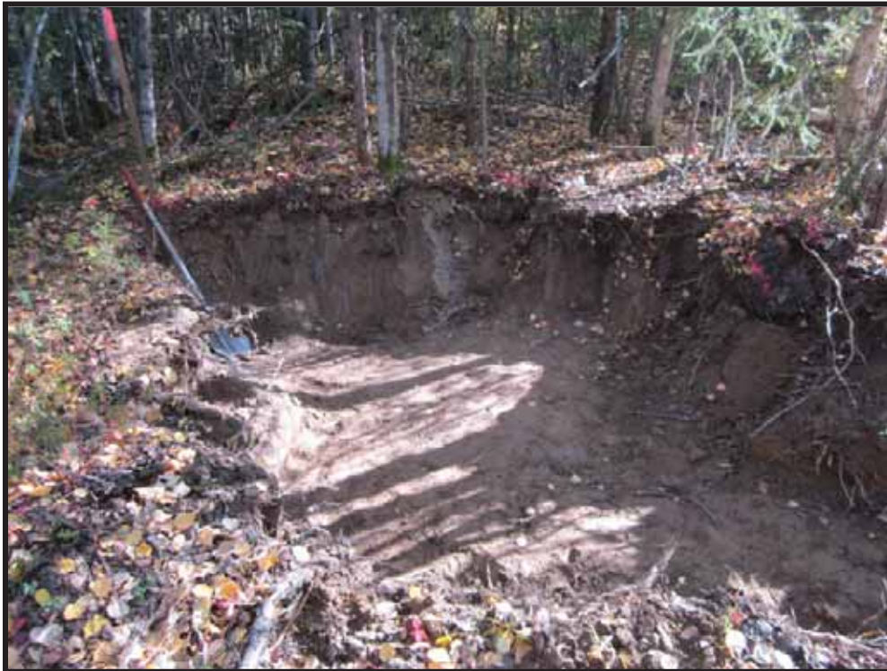
Photo 3: Looking southeast after September 2012 excavation.
