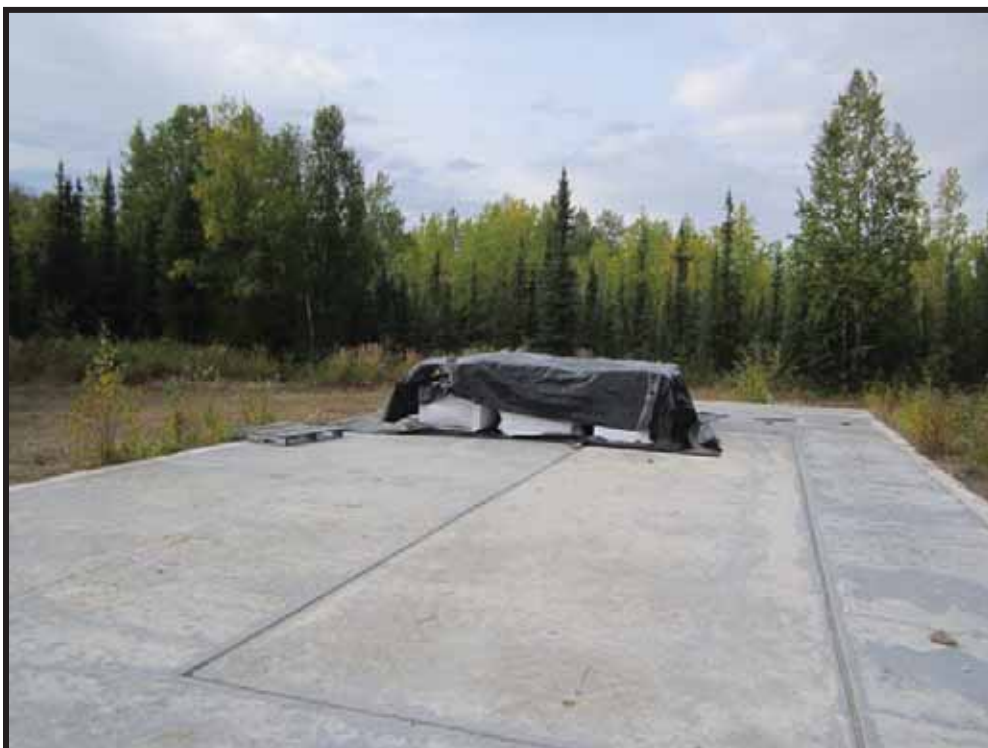
Photo 8: Mercury contaminated soils containerized in cubic yard boxes for disposal.
