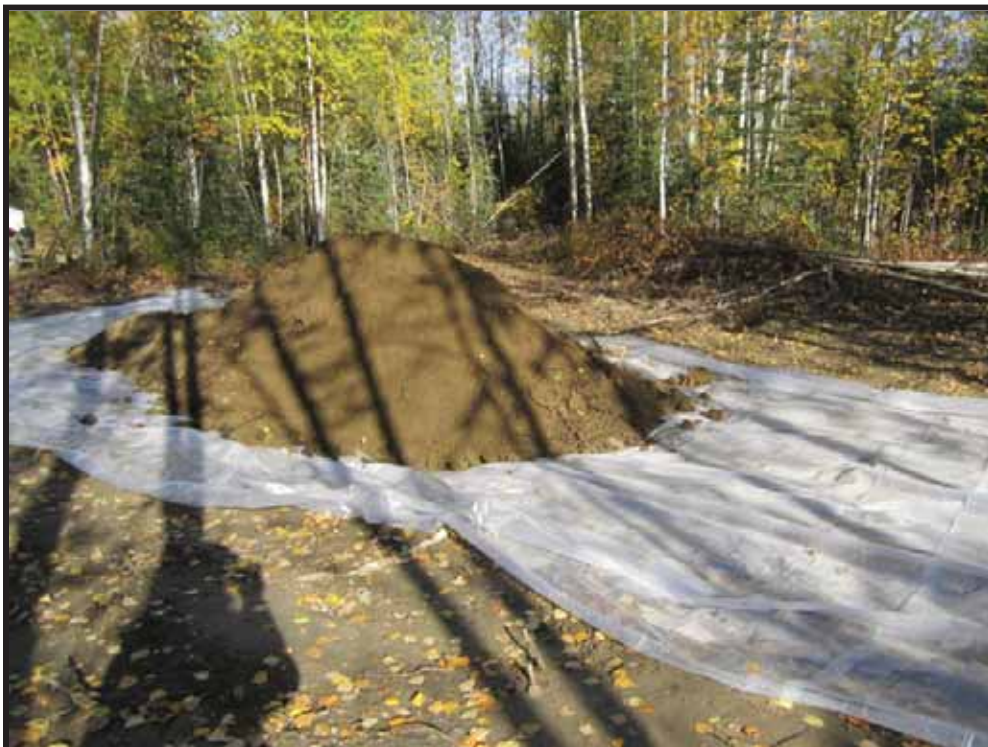
Photo 4: Typical stockpile construction with reinforced polyethylene liner and cover.
