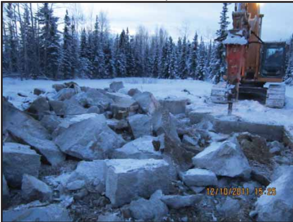
Photo 5: Concrete foundation during mechanical demolition.
