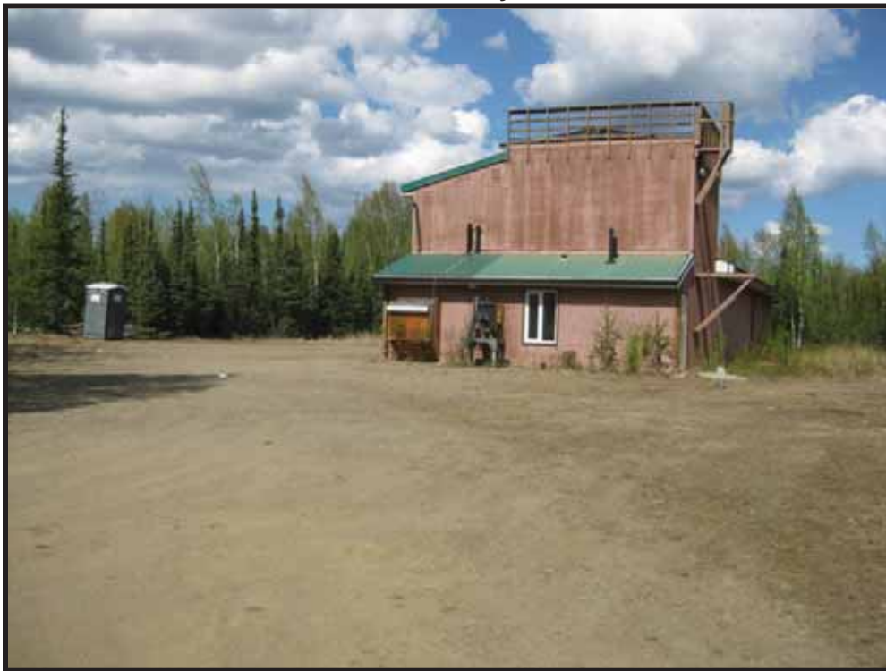
Photo 1: LIDAR Tower site containing Liquid Mirror Telescope (LMT).
