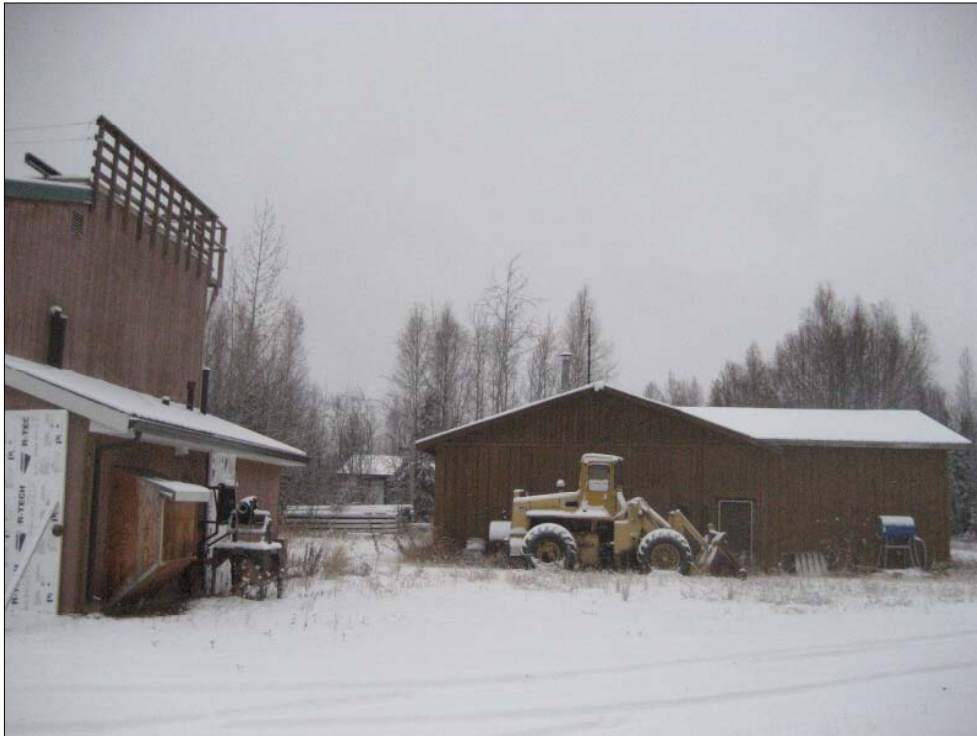
Photo 27 - Looking east across the front of the LIDAR Building at the west side of the Garage/Shop with fuel drum and heating oil tank visible
