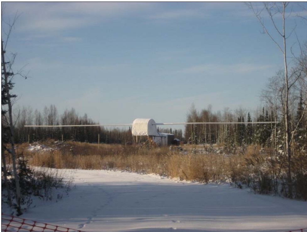
Photo 34 - Looking west at the more recent Dipole Antenna and associated structure, that includes a heating oil storage tank located to right of the small building
