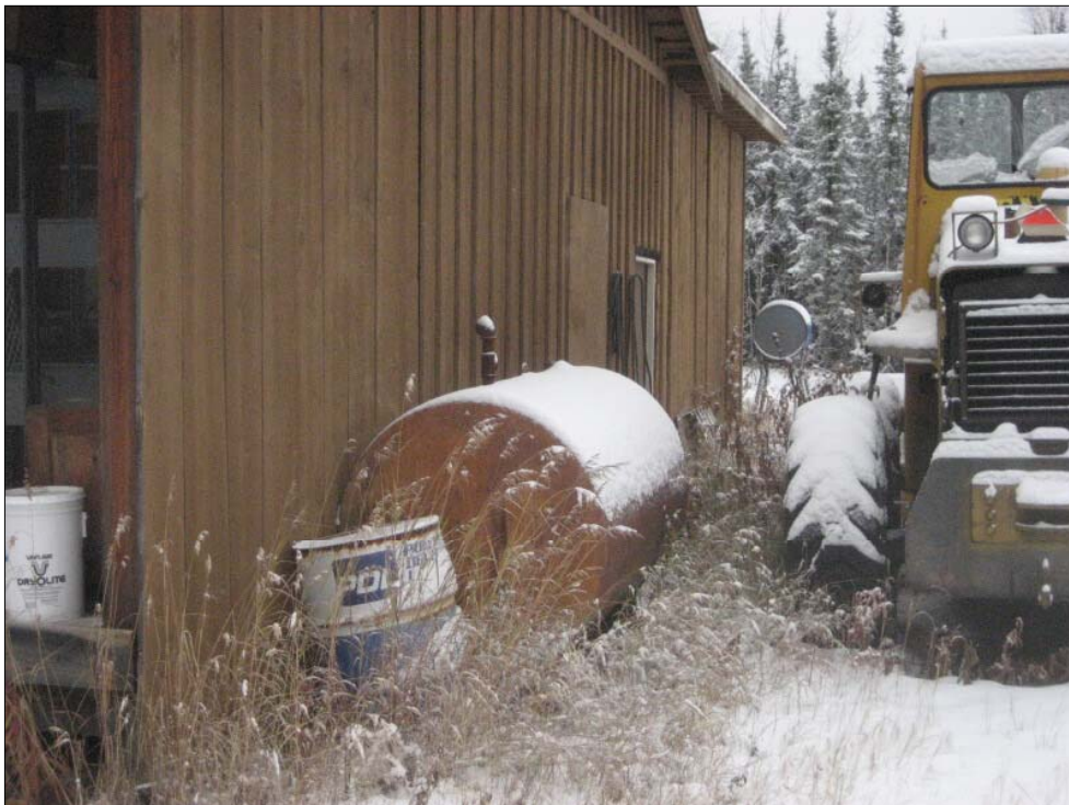
Photo 28 - Detail view of heating oil tank on west exterior wall of Garage/Shop with fuel dispensing drum in background
