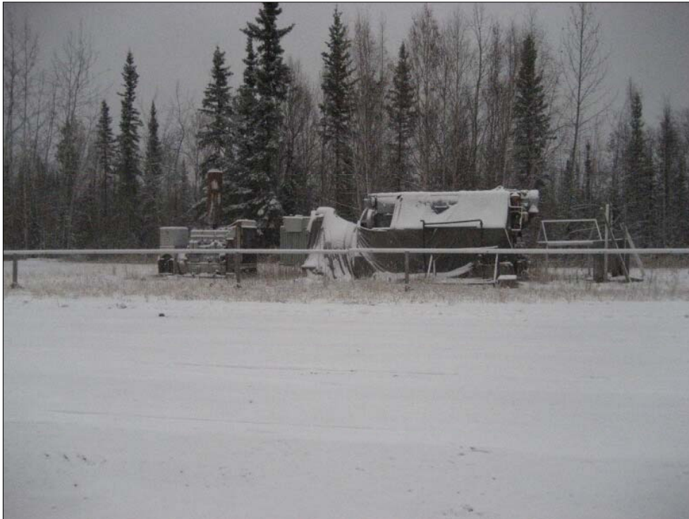
Photo 03 - Unused generators stored to south of the Generator Building; smaller unit has been removed from the Site
