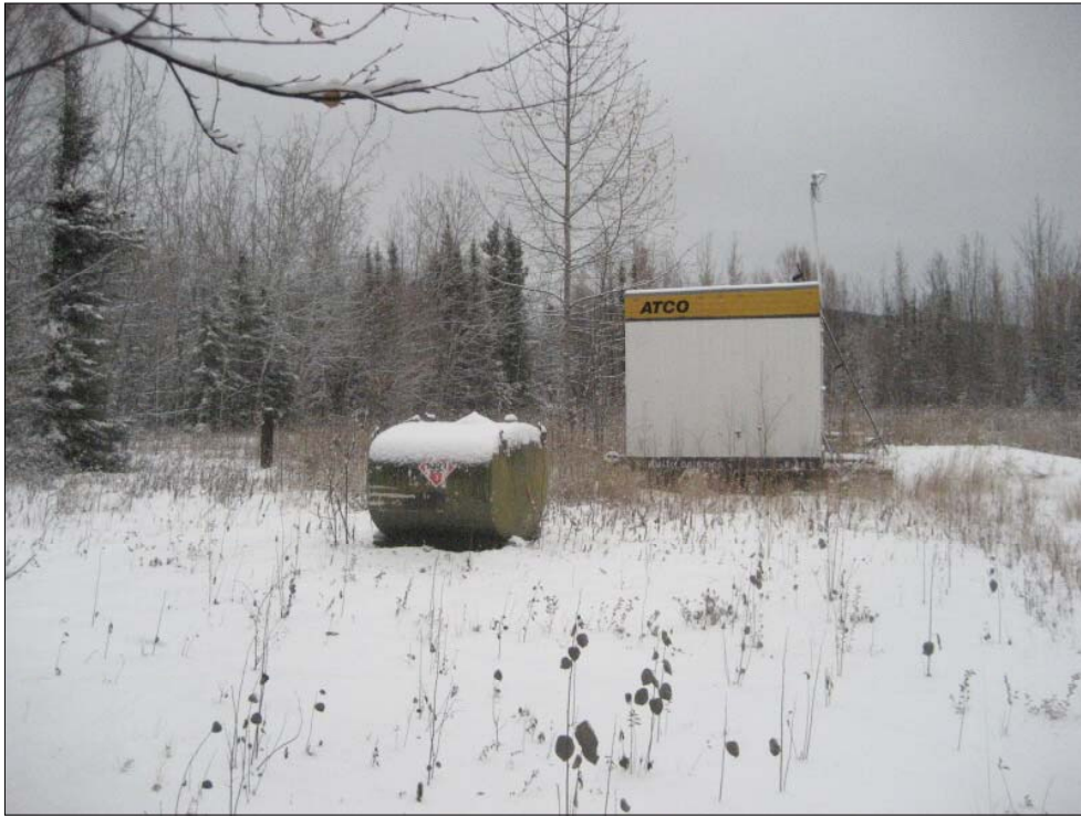
Photo 33 - Looking south at the ATCO unit and associated fuel storage tank
