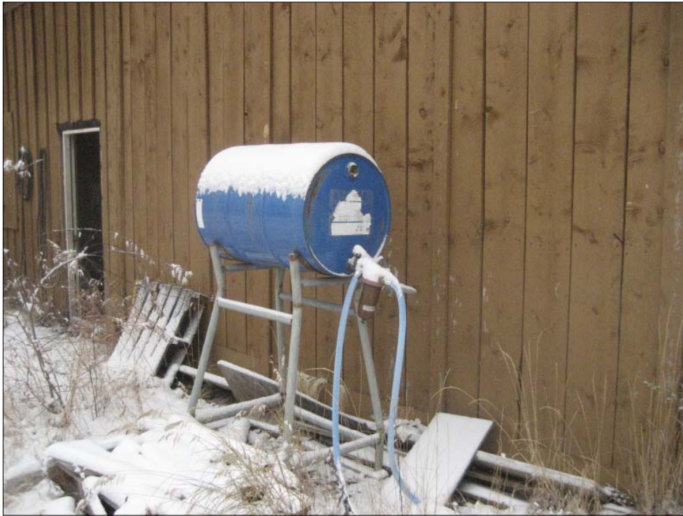
Photo 29 - Drum used as gasoline fuel dispenser along west exterior wall of Garage/Shop
