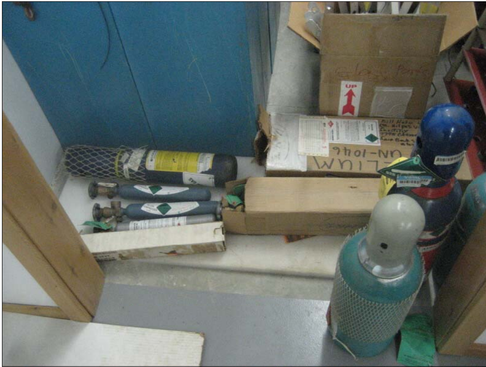
Photo 21 - Gas cylinders of various size and content located inside the LIDAR Building; several of the larger tanks have been removed while smaller tanks remain in the building
