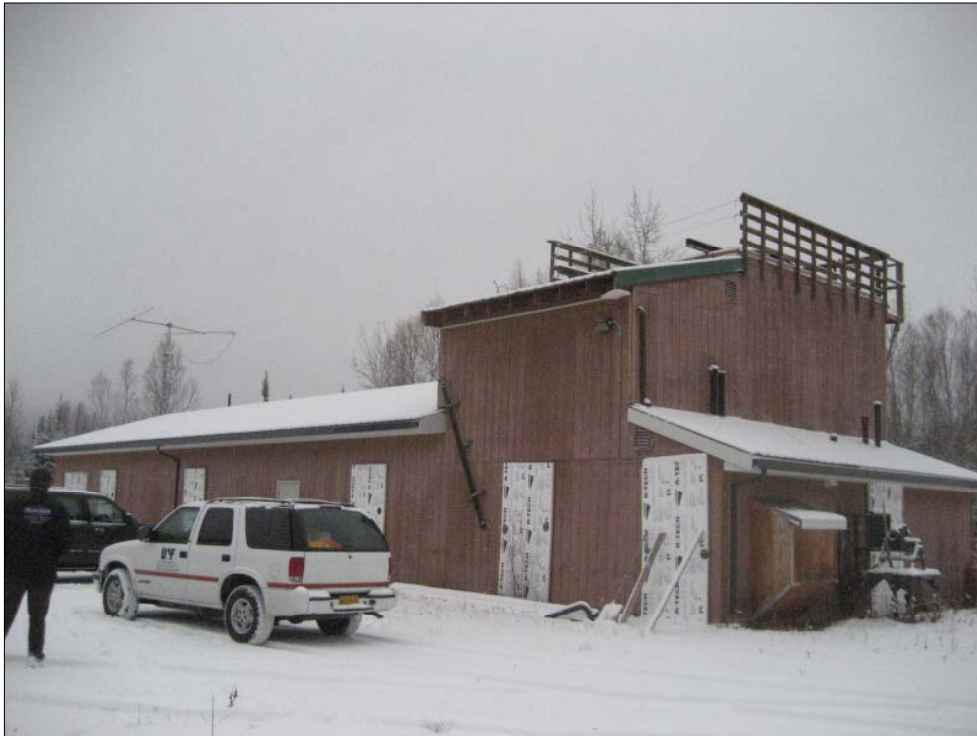
Photo 19 - Looking northeast at the exterior of the LIDAR Building
