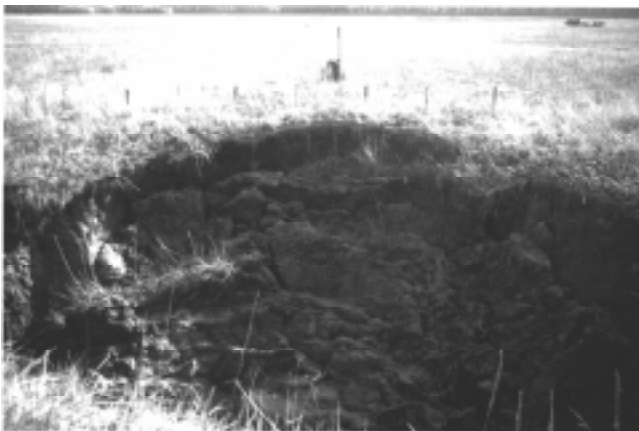
Figure 9. Headwall erosion study site. The line of stakes approximately parallels the gully crest. The hub stake is to the right of center behind the stake line.
