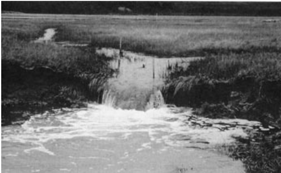
Figure 57. Water flowing over gully headwall at Parachute Gully plunge pool.
