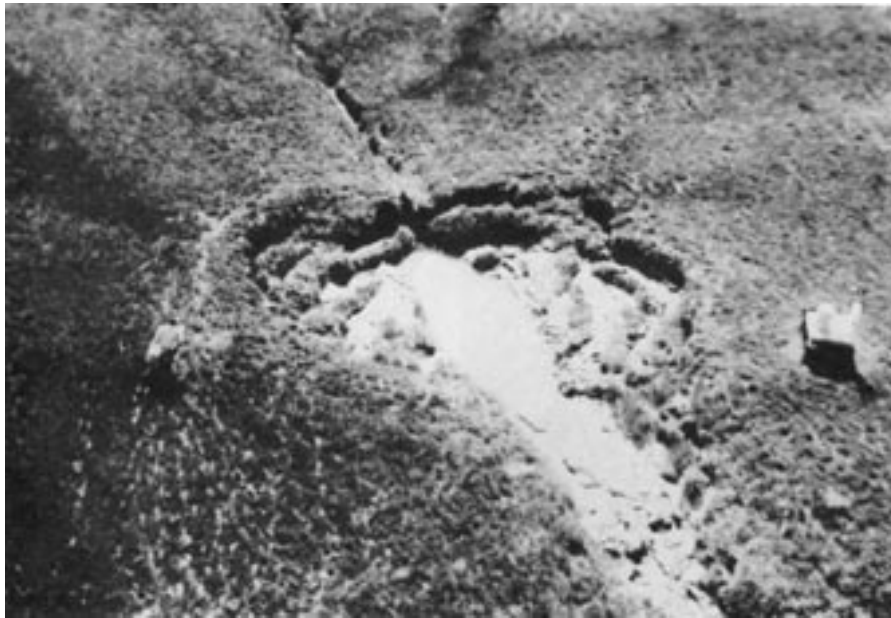
a. Plunge pool of Mortar Gully.
