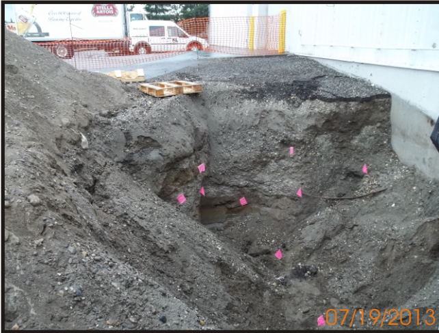
Photograph 1: Subject property after excavation - viewed northwest
