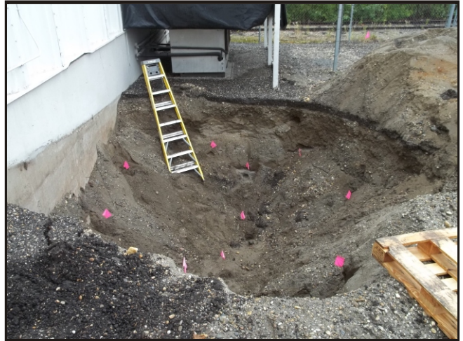
Photograph 2: Subject property after excavation - viewed east
