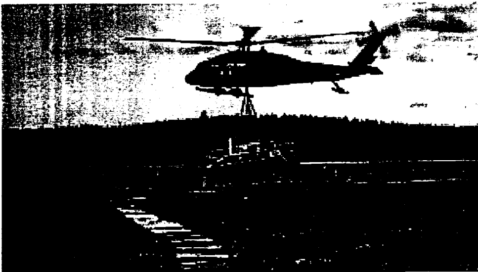
Figure III-4-8. Airlifting the genset into place using a UH-60 Blackhawk helicopter.
