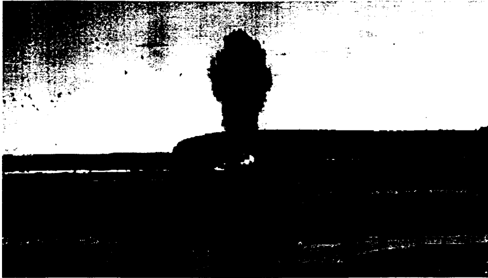
Figure III-4-6. Blasting of the sump using two 40-lb cratering charges.
