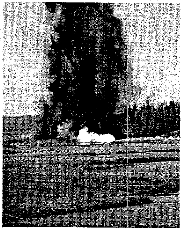
Figure III-1-2. Blasting of sump for Pond 146.
