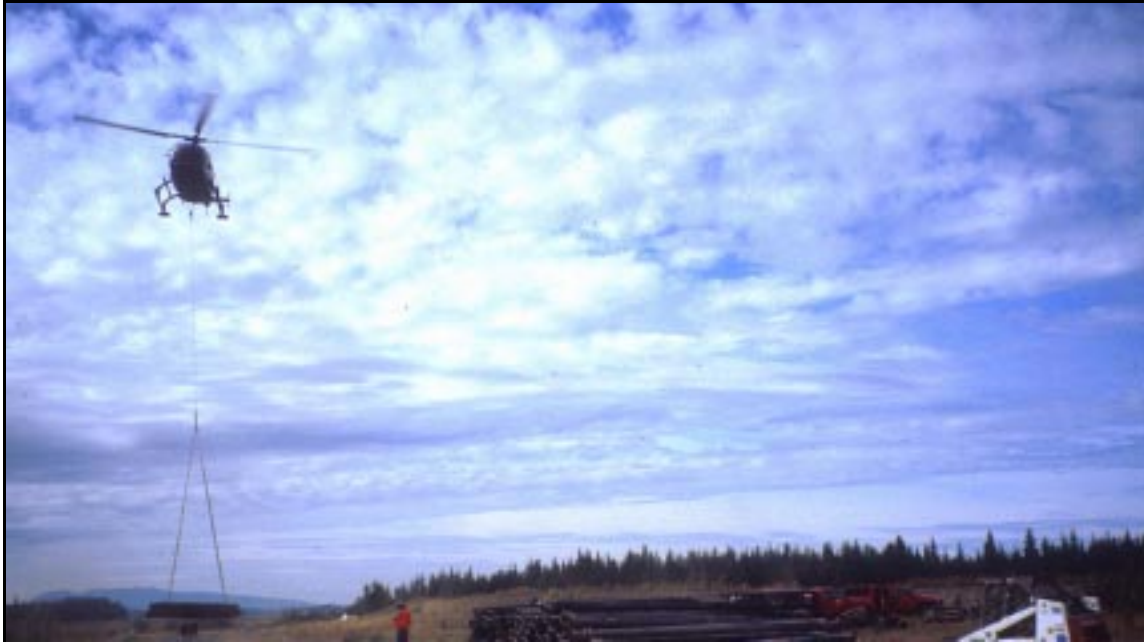
Figure III-1-3. Retrograde of pipe to EOD Pad using slings.
