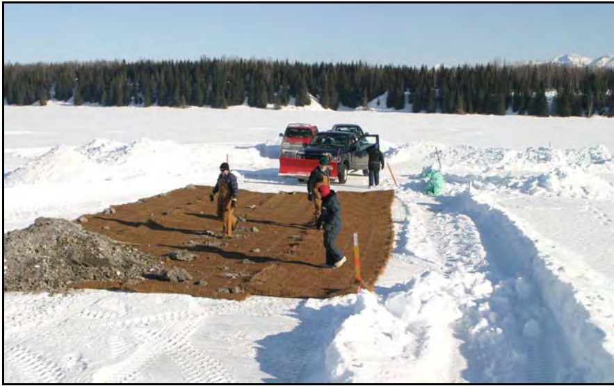
a. Laying out geotextile mat at test site. Note survey markers.
